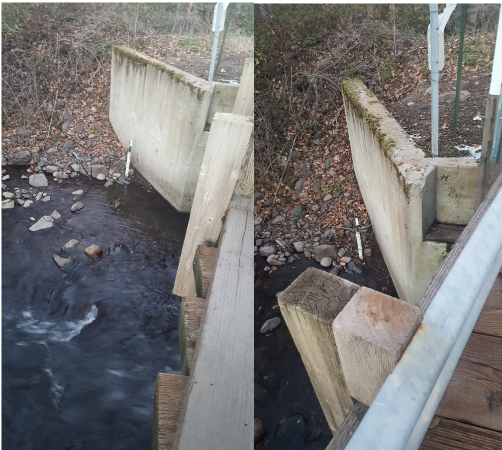
Figure 3. Water Level Gauge in Shovel Creek at Bridge on Ager Beswick Road
