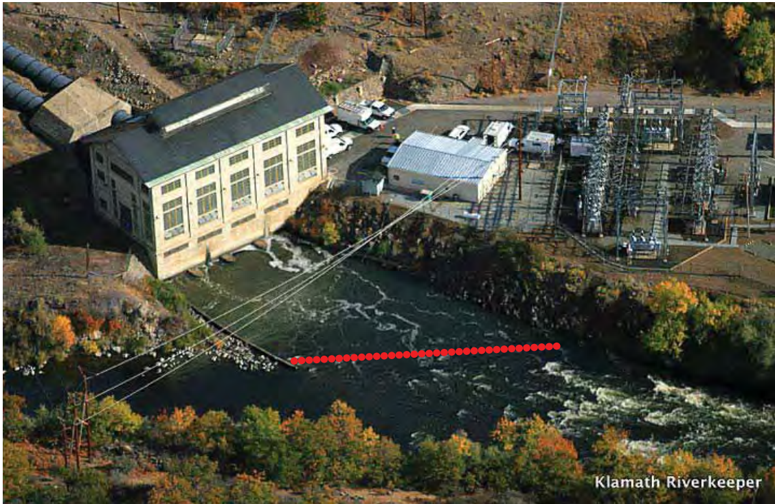
Figure 2-26. Modifications at the tailrace of the Copco 2 Powerplant would extend the bank and install a tailrace barrier screen (red dots).
