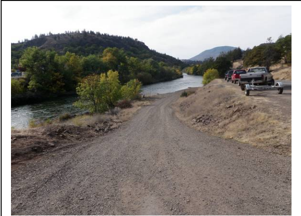
R.1.5-1: Iron Gate Boat Launch (CDM 2010)
