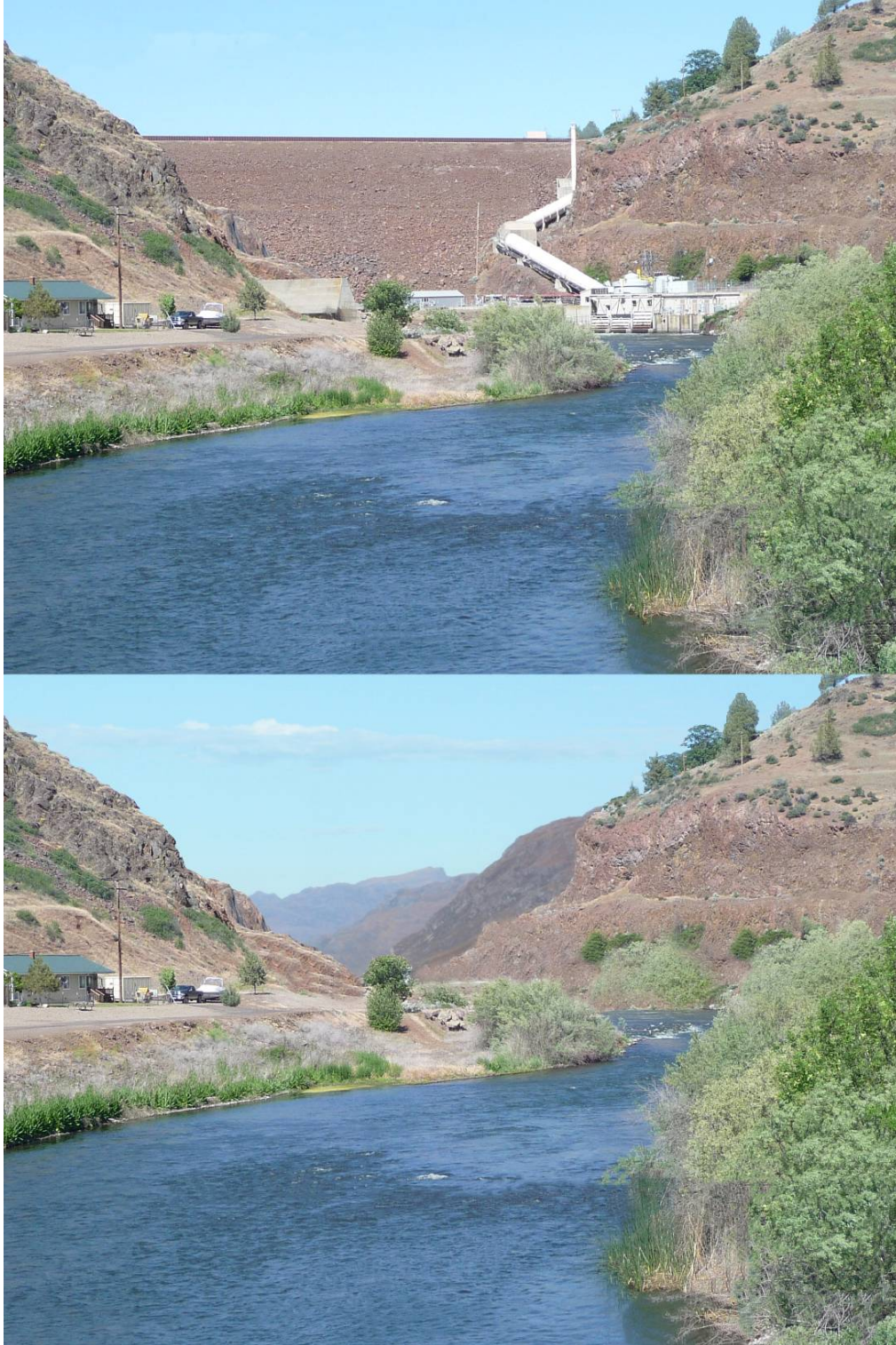
Figure 3.19-9. Iron Gate Dam Before Removal (top) and a Simulation of What the Facility Could Look Like After Dam Removal (bottom) Except for Landform/Vegetation Restoration Details Which Were Not Known at the Time of Simulation. Note that the residence shown in the foreground would also be removed under the Proposed Project Source: 2012 KHSA EIS/EIR.
