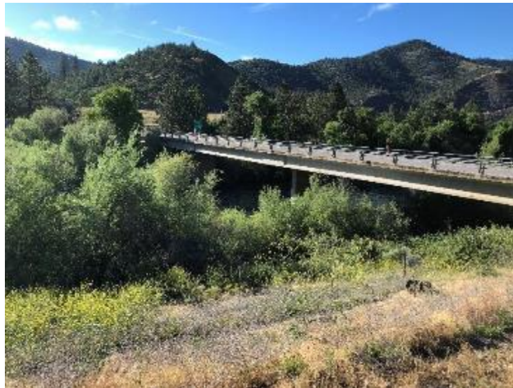
Figure IND46-ORAL1-2. Klamath River Bridge 2-135 (June 5, 2019).
