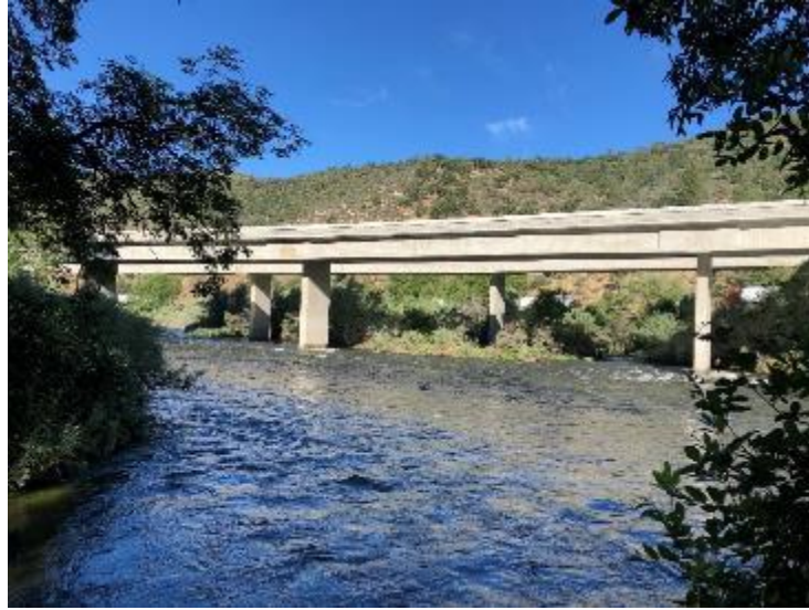
Figure IND46-ORAL1-1. Klamath River looking downstream at the Interstate 5 Bridges (June 5, 2019).
