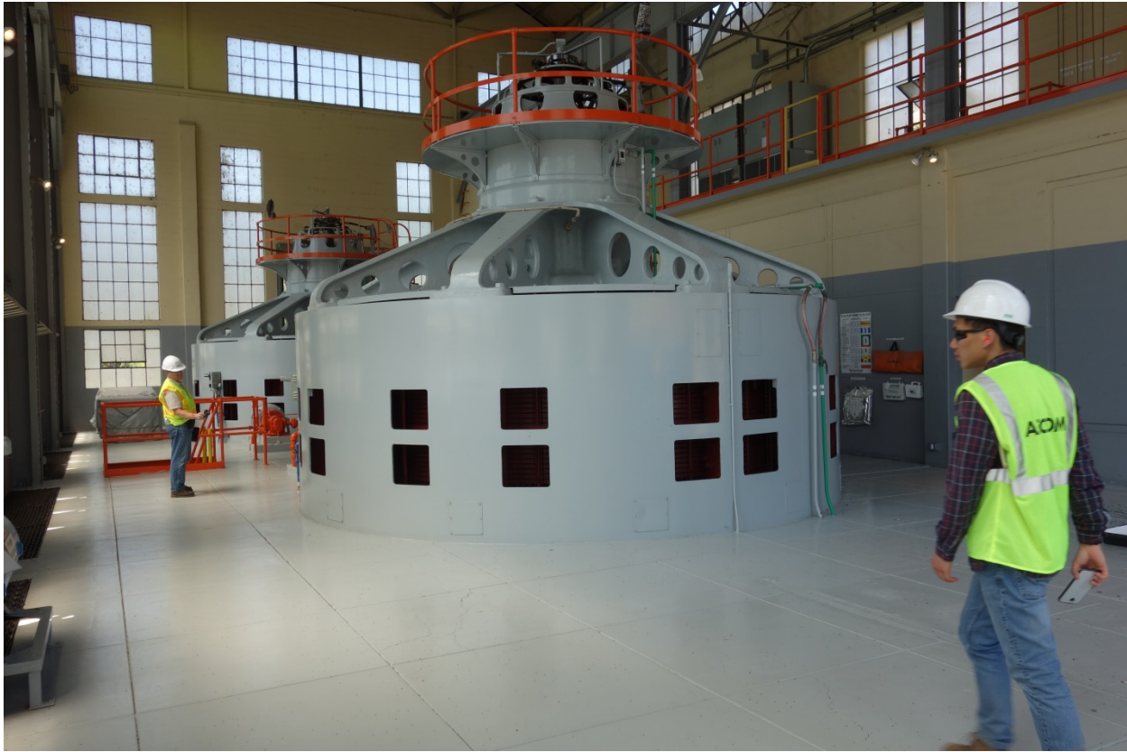
Figure 2.3-7 Copco No. 2 Powerhouse
