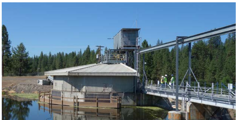
Figure 2.1-6 J.C. Boyle Intake Structure
