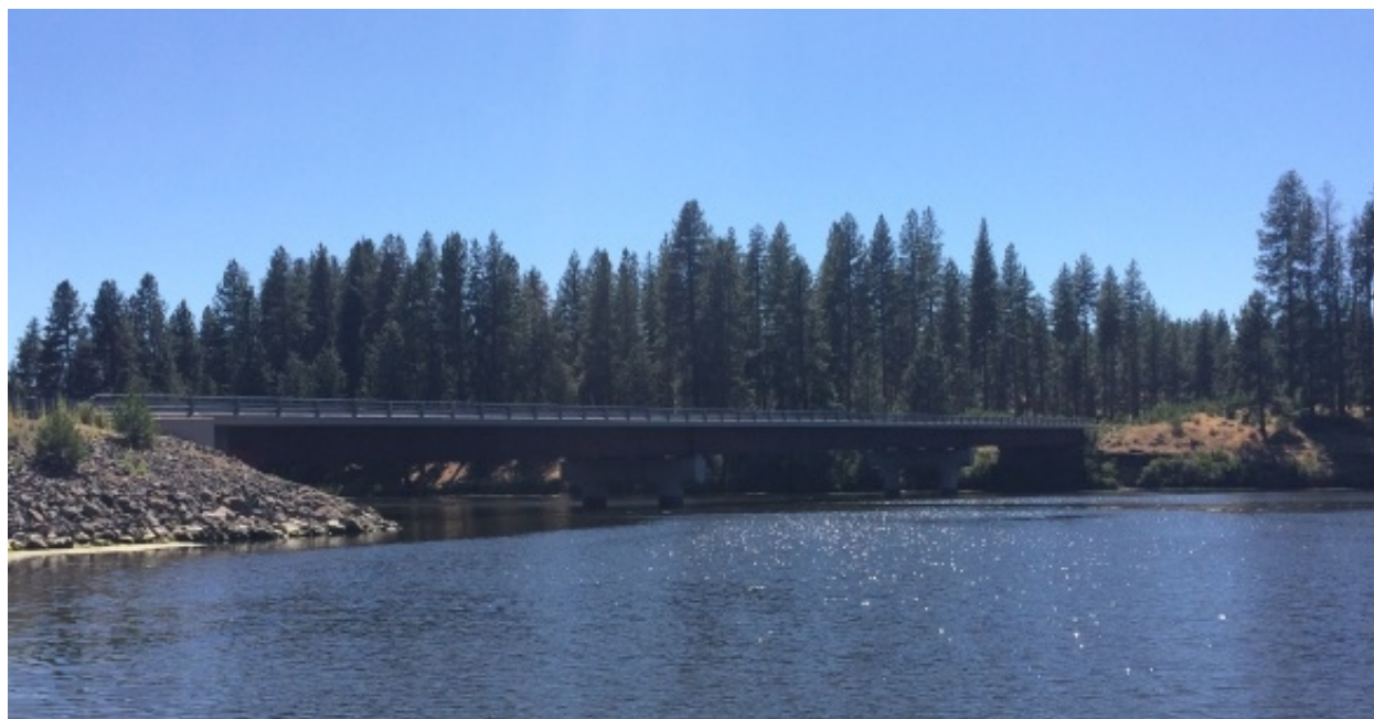
Figure 5.2-3 Spencer Bridge (OR66)
