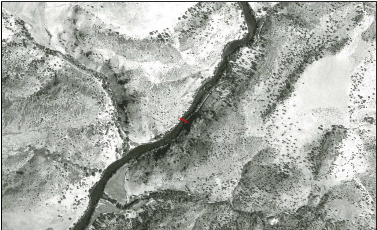
Figure 2-12 Aerial photo of Iron Gate Dam location prior to construction in 1955
