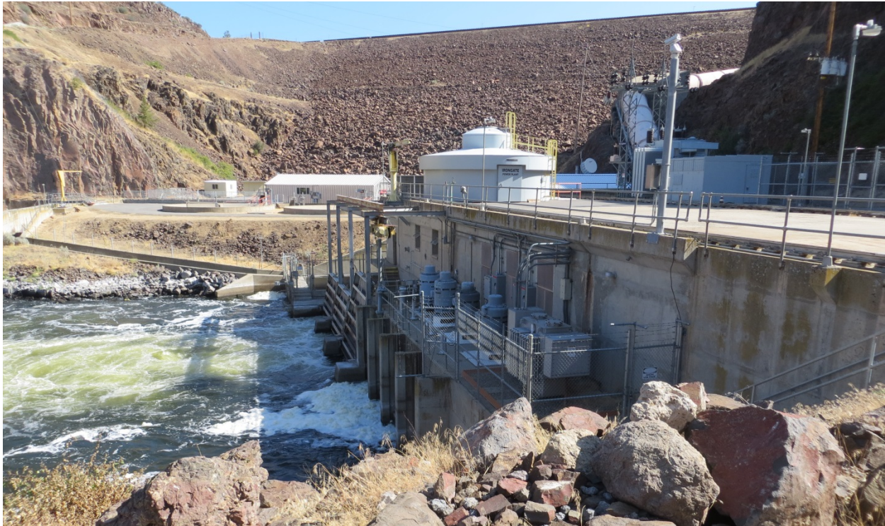
Figure 2.4-6 Iron Gate Powerhouse
