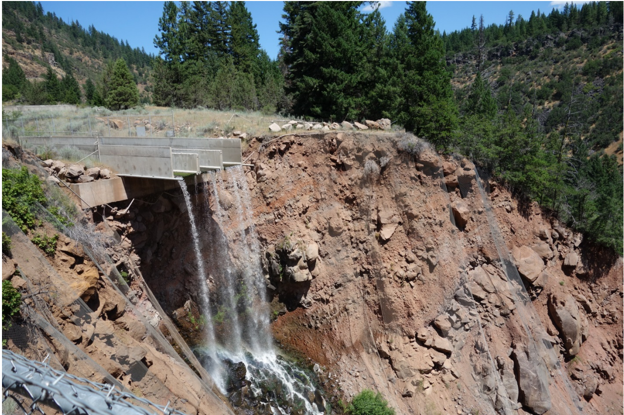
Figure 2.1-8 Forebay Overflow Chute and Upper Portion of Scour Hole
