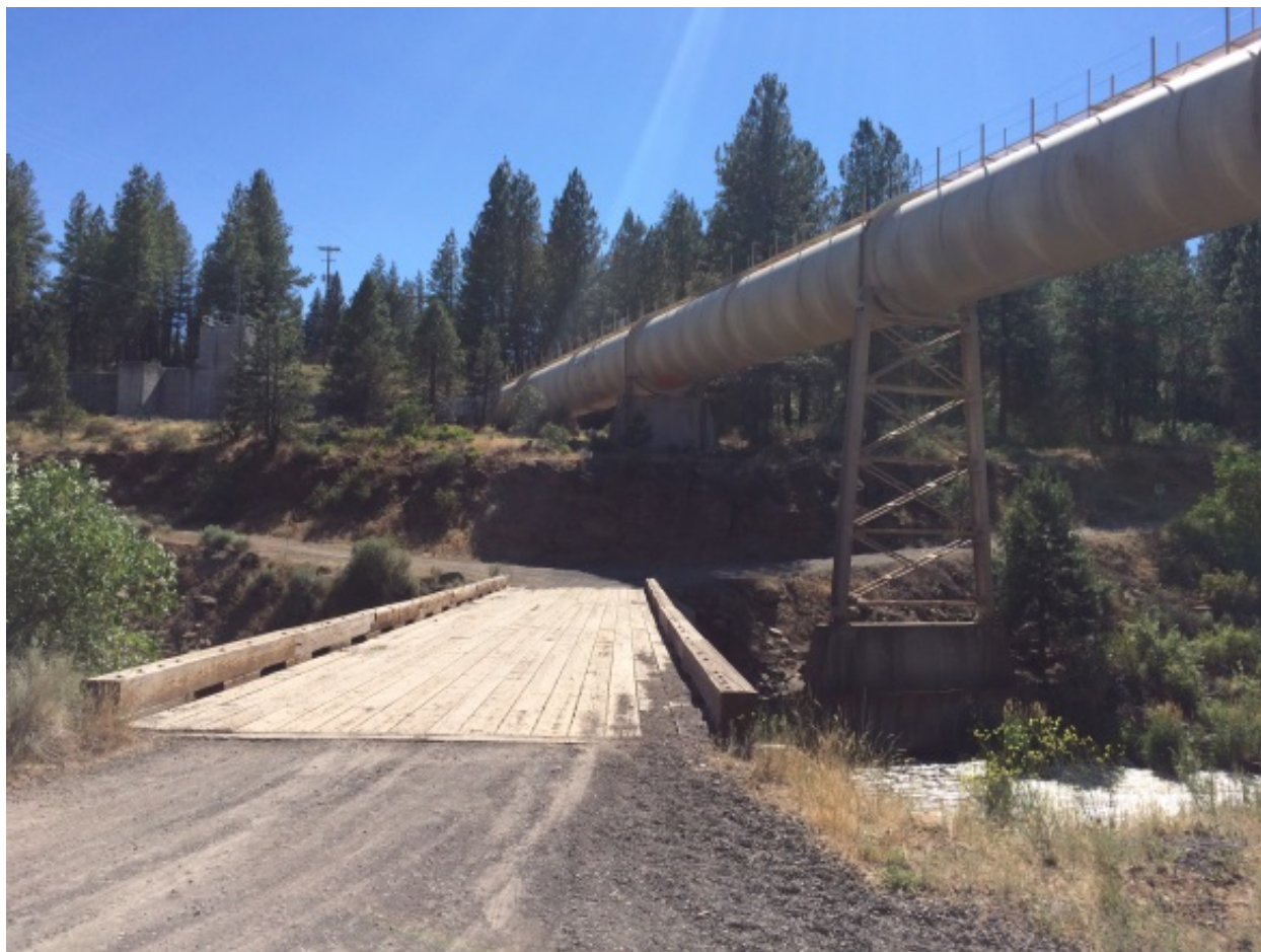
Figure 5.2-5 Timber Bridge at J.C. Boyle
