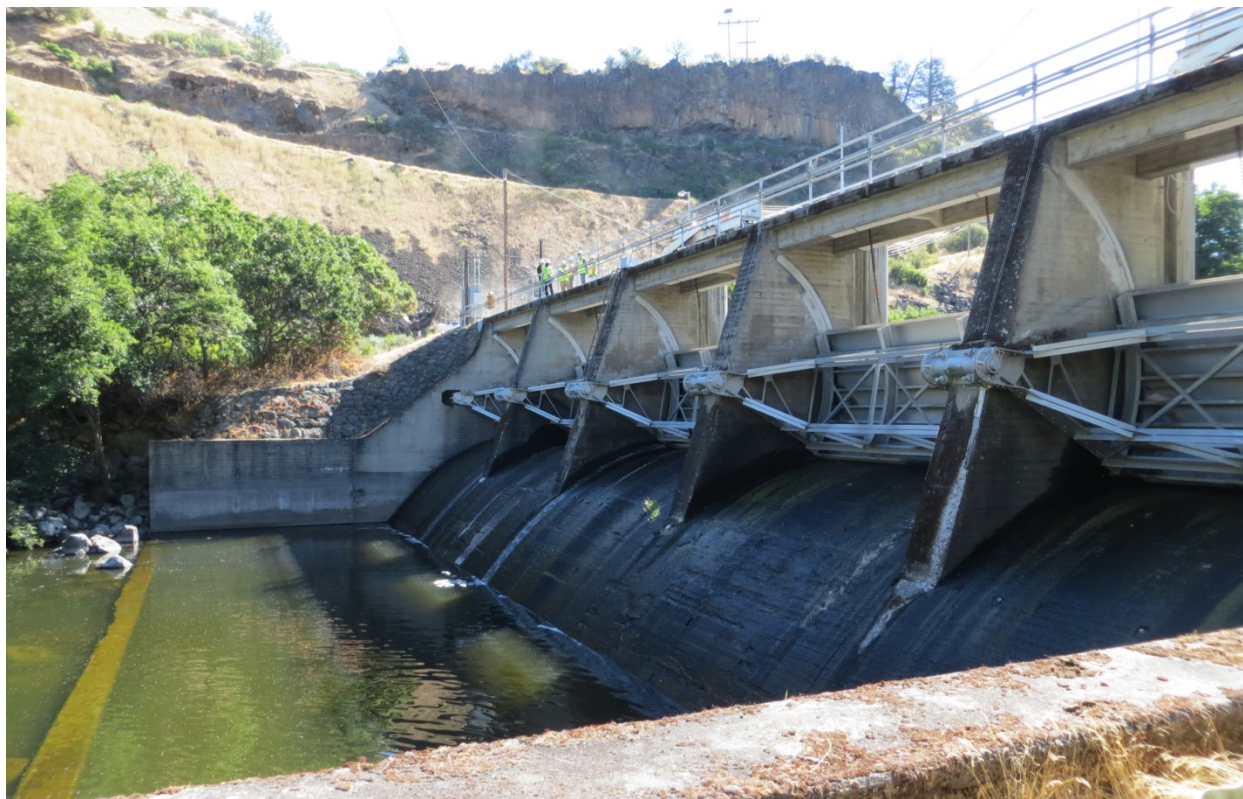
Figure 2.3-1 Copco No. 2 Dam from Downstream Side
