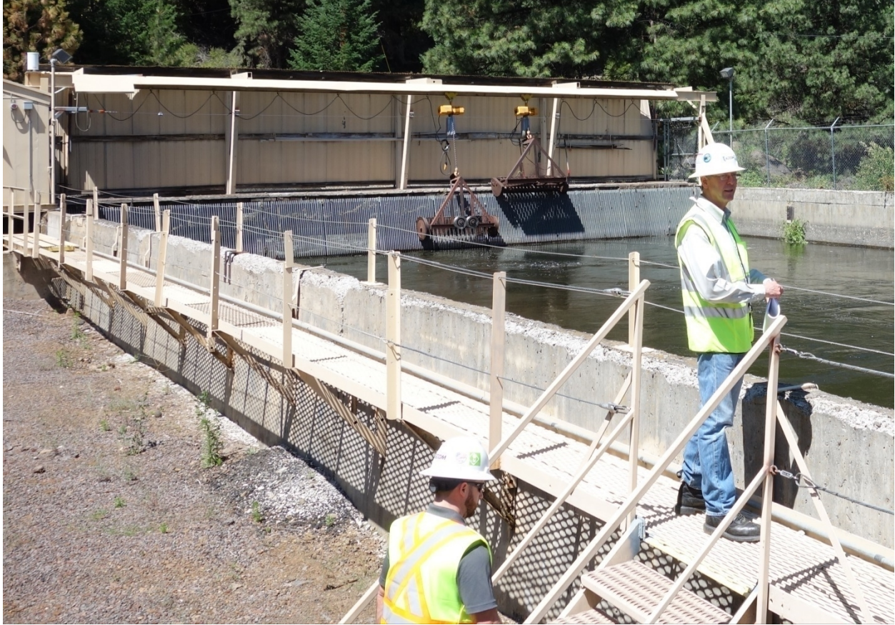
Figure 2.1-9 J.C. Boyle Forebay and Tunnel Trash Rack (left)
