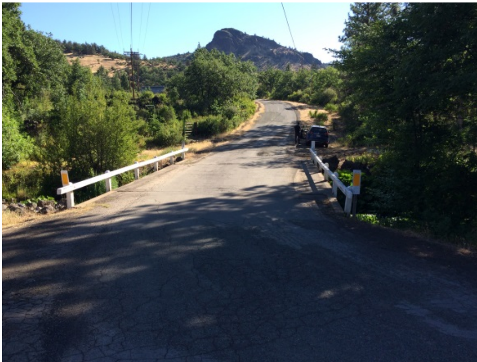
Figure 5.3-4 Fall Creek Bridge on Copco Road
