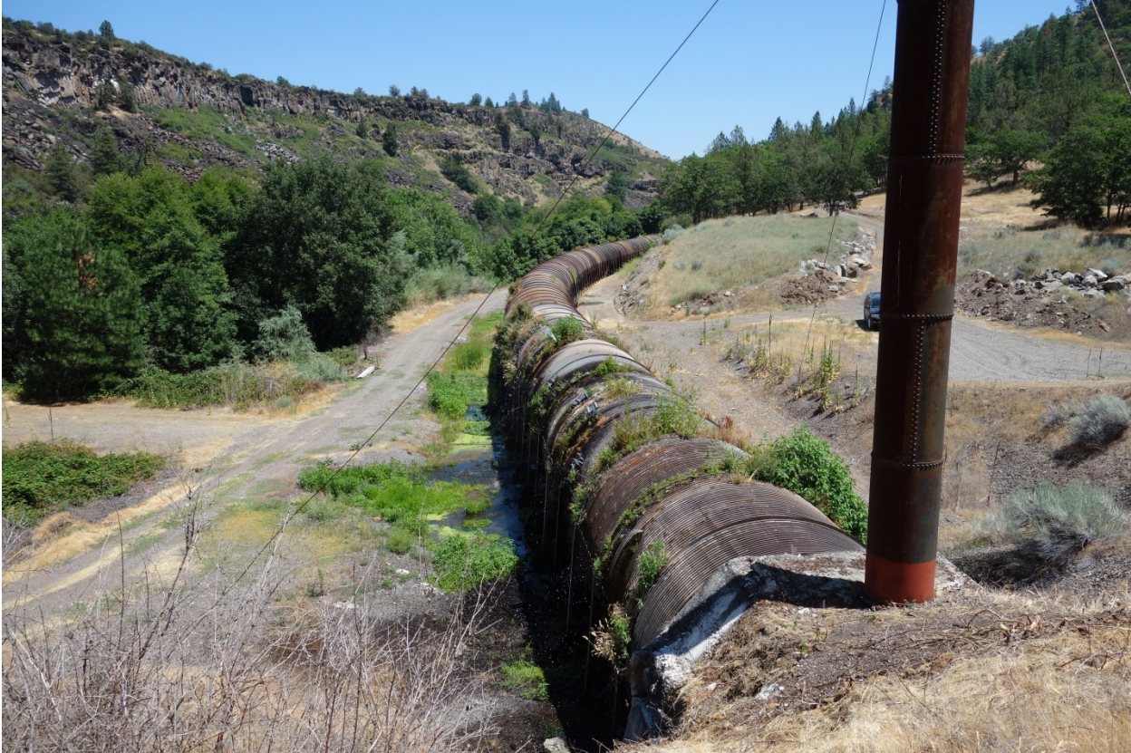
Figure 2.3-6 Copco No. 2 Wood-Stave Penstock
