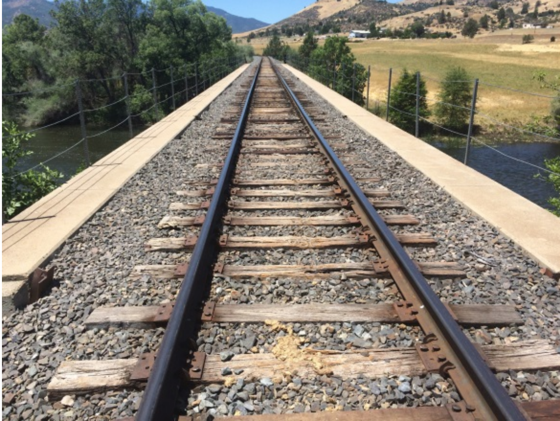
Figure 8.1-3 Rail Road Bridge
