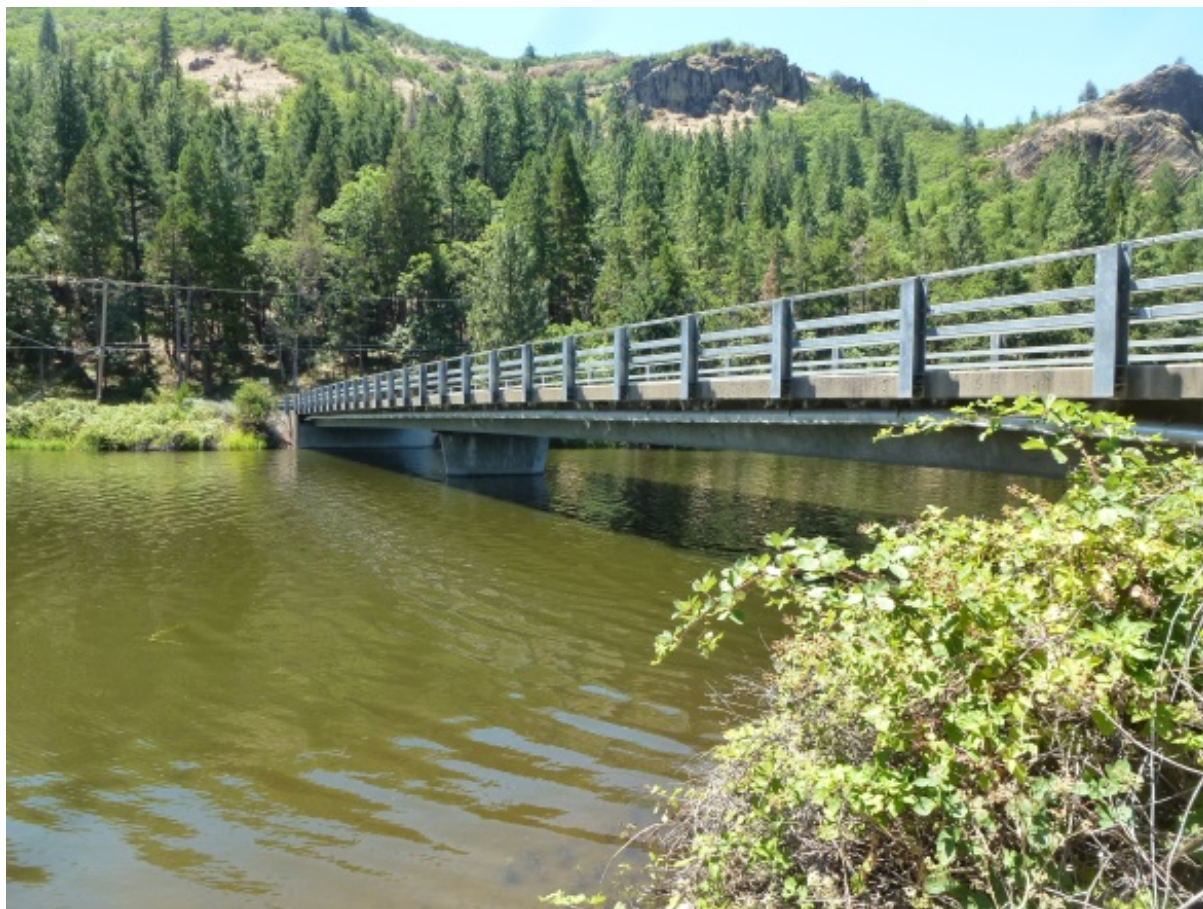
Figure 5.3-6 Copco Road Bridge
