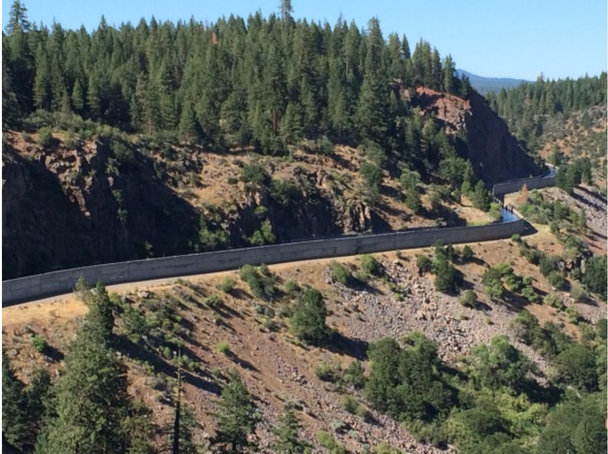
Figure 5.2-6 Power Canal Access Road
