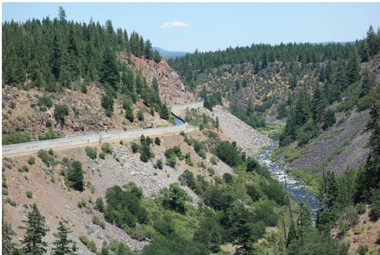
Figure 2.1-7 J.C. Boyle Power Canal (left) and Klamath River Bypass Reach (right)
