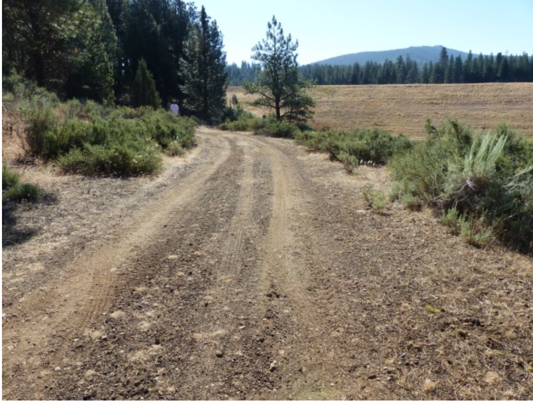
Figure 5.2-7 Right Abutment Access Road
