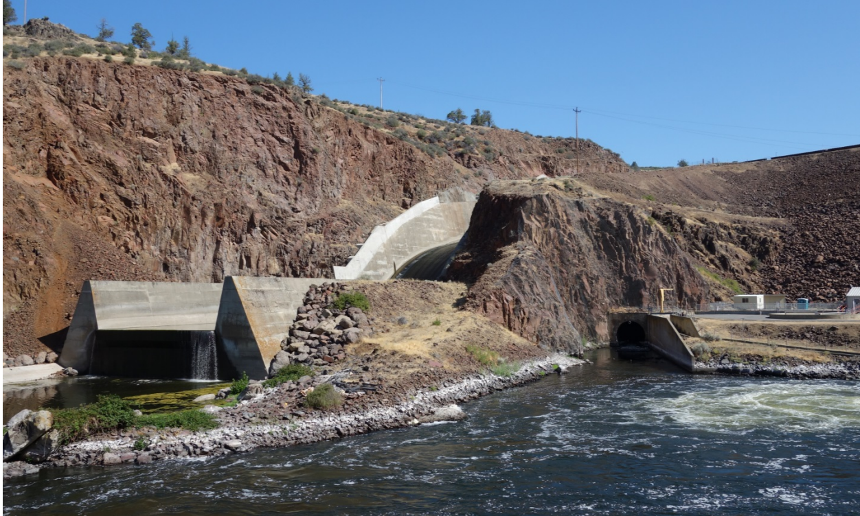
Figure 2.4-5 Iron Gate Diversion Tunnel Outlet (center-right, in shadow)
