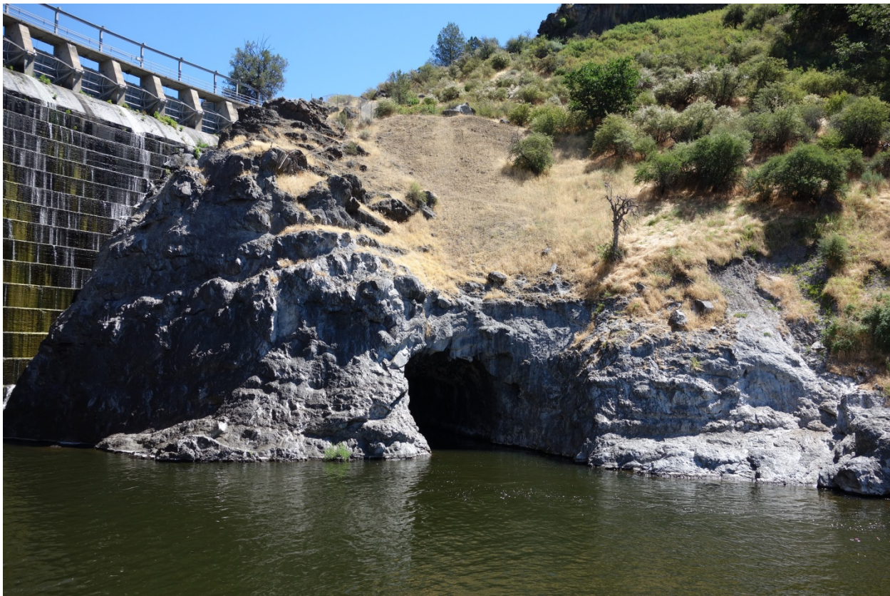
Figure 2.2-5 Copco No. 1 Diversion Tunnel Downstream Portal
