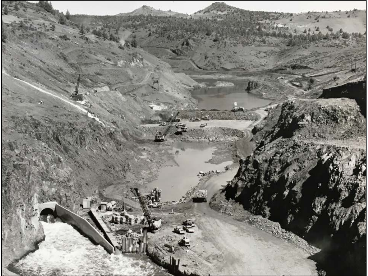
Figure 2-13 Photo of Iron Gate Dam during construction and showing reservoir area
