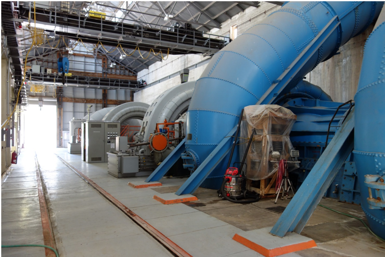
Figure 2.2-7 Copco No. 1 Powerhouse
