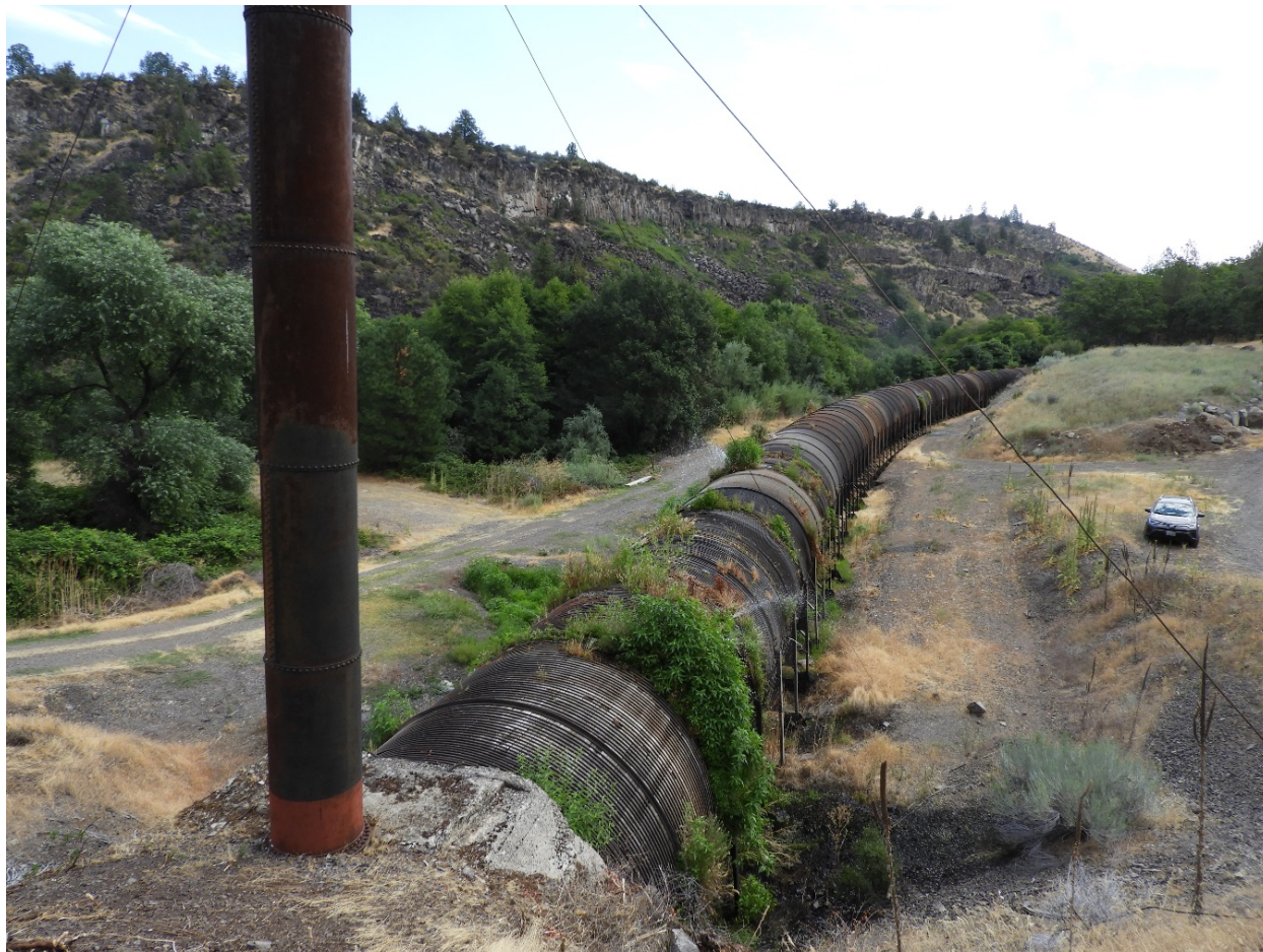
Figure 3.4-6 Copco No. 2 Penstock
