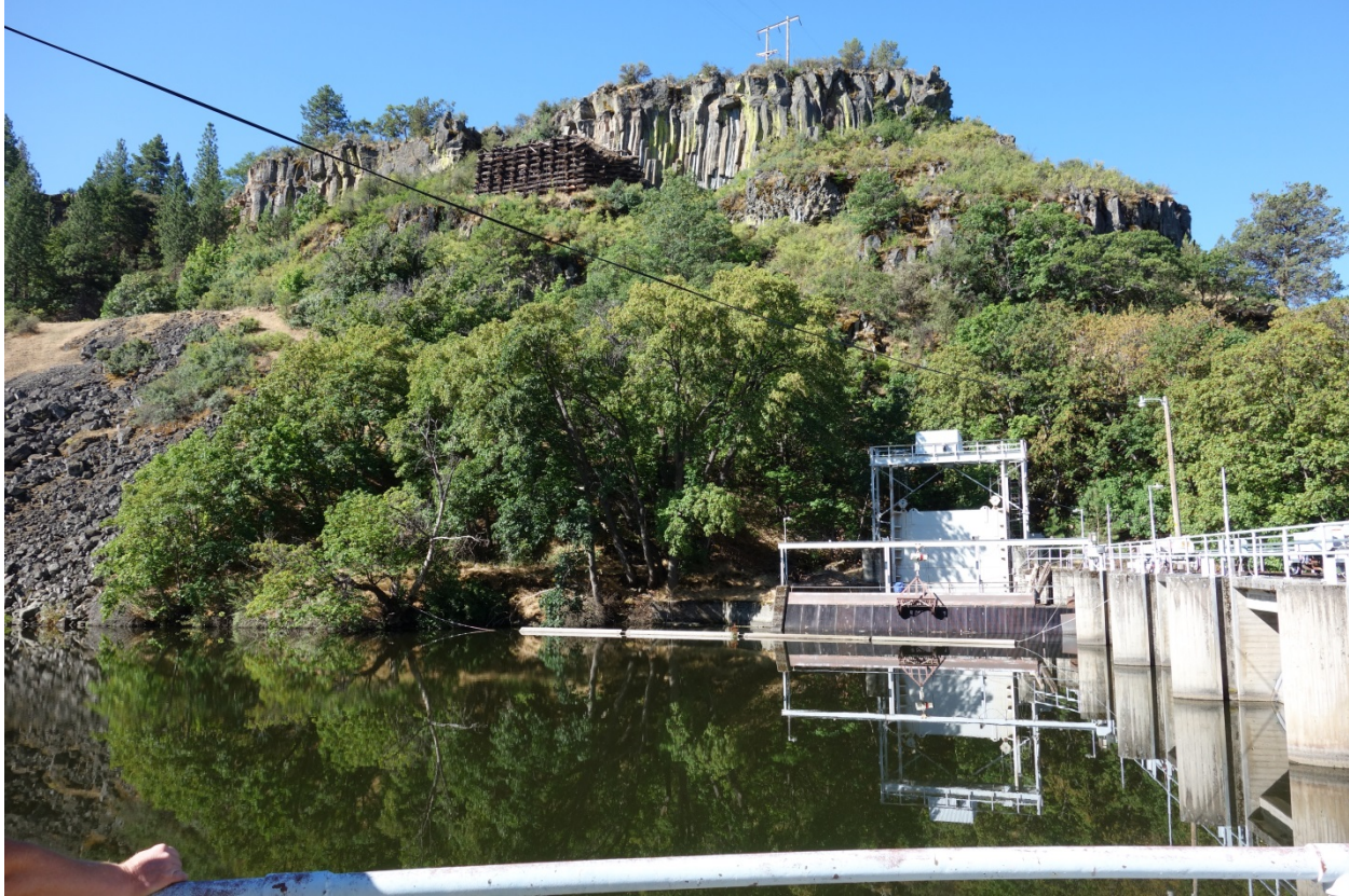
Figure 2.3-5 Copco No. 2 Dam from Upstream Side Showing Intake (at water level) and Crib Wall (high) on Left Abutment
