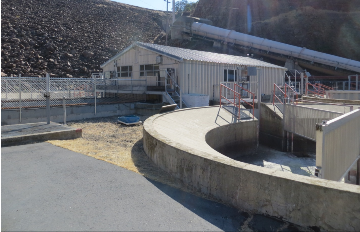
Figure 2.4-7 Iron Gate Fish Holding Tanks and Spawning Building
