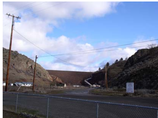
Iron Gate Dam 2
