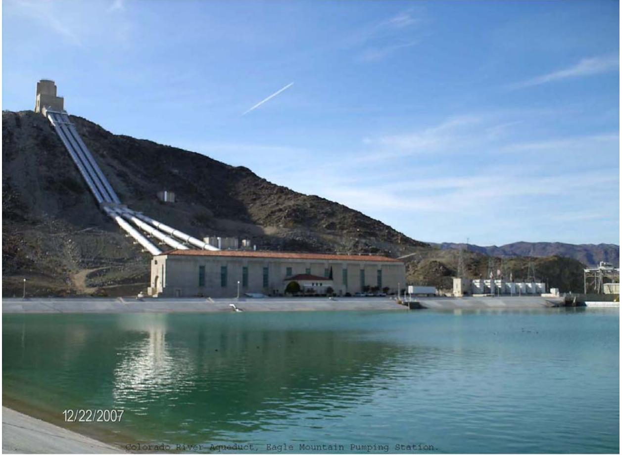
Photo 9. Photo of the Colorado River Aqueduct pumping station (1 of 2). Photo taken in 2007.
