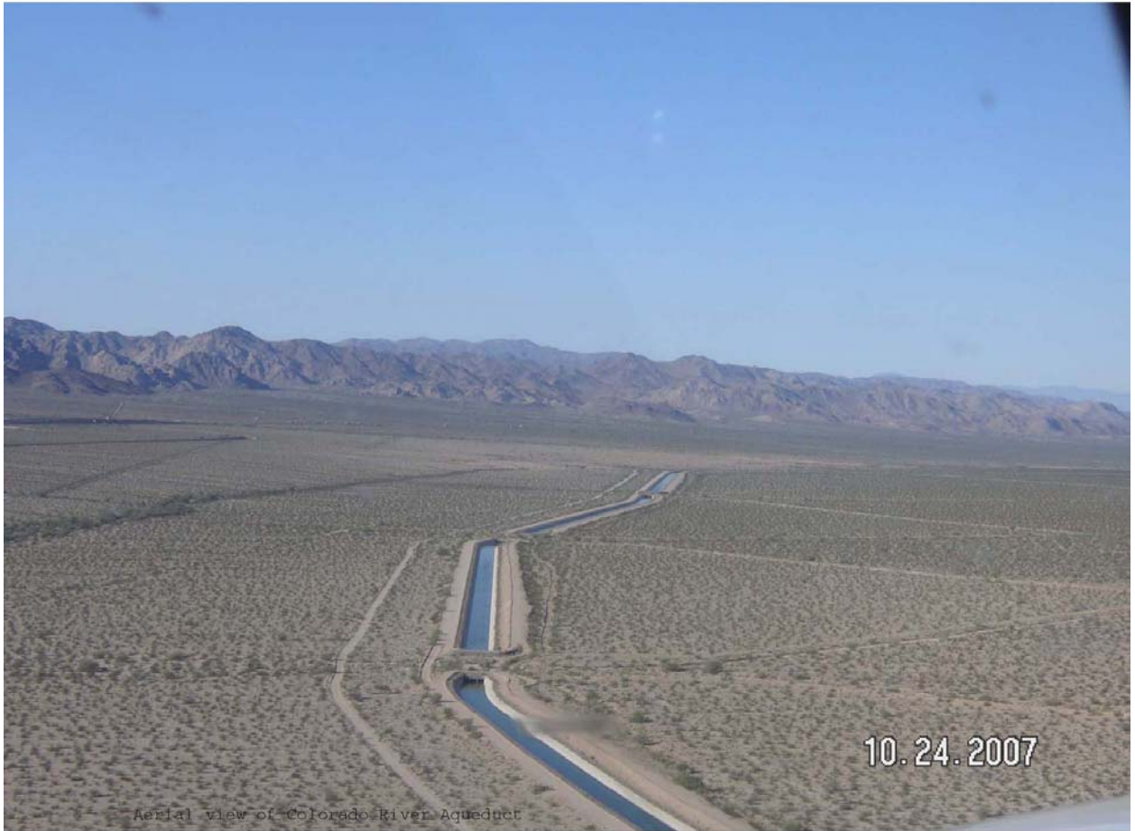
Photo 8. Photo of open air segment of the Colorado River Aqueduct. Photo taken in 2007.
