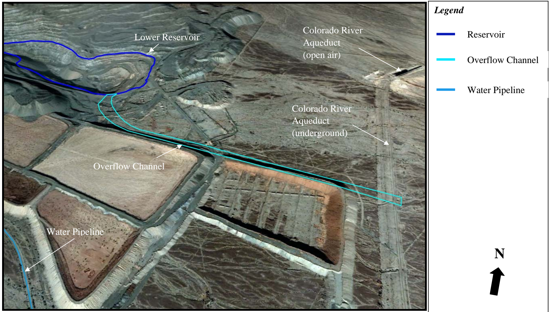
H-4. Simulated view the Lower Reservoir and overflow channel from approximately 1200 feet, facing north (Source: Project Plan from ECE, aerial imagery and 3D simulation from Google Earth, 2011 imagery, as modified by staff)
