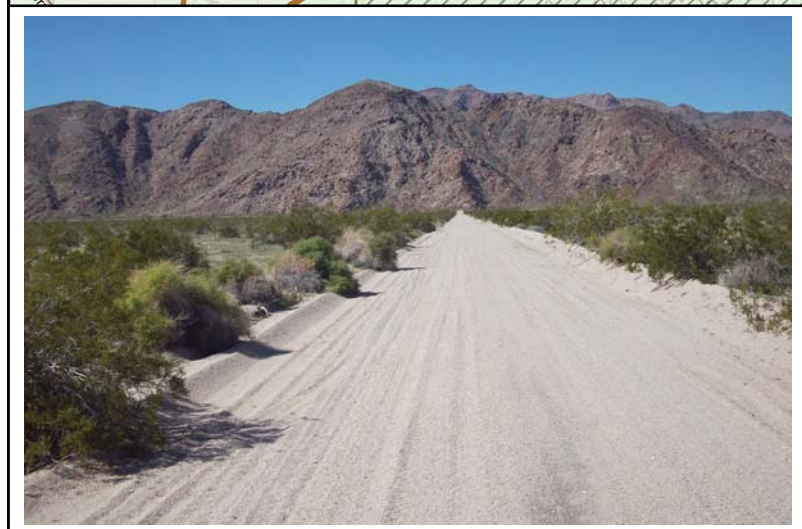
Typical Maintained Dirt Road
