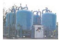
Well-head treatment facilities to remove water contamination.
