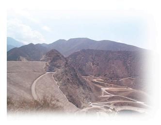
Floodwaters slowed by Seven Oaks Dam (in the left of this picture) would be diverted at either the plunge pool (lower right of picture) or Cuttle Weir. New facilities would be built near the plunge pool, and captured water would be conveyed in new and existing facilities for use in the Muni and Western service areas.
