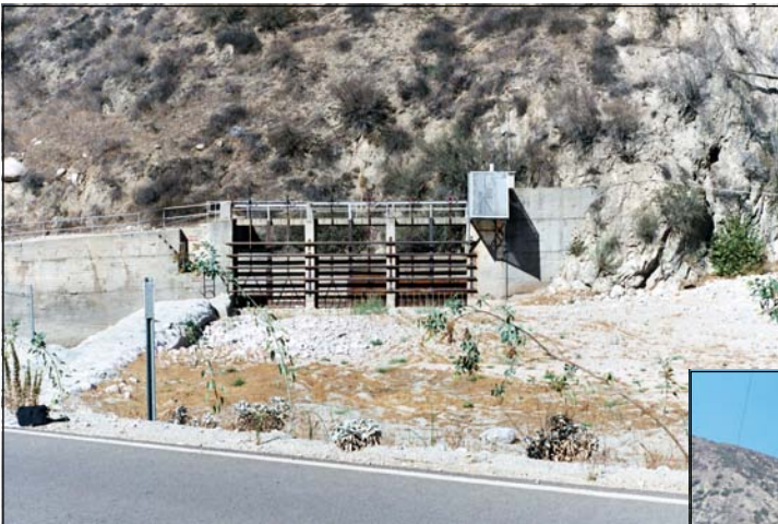
Francis Cuttle Weir Dam and Associated Diversion Structure
