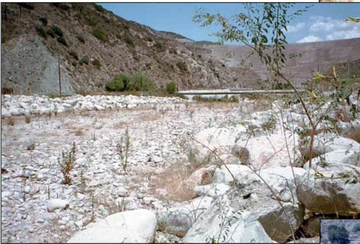
Section of the North Fork Canal Crossing the Santa Ana River
