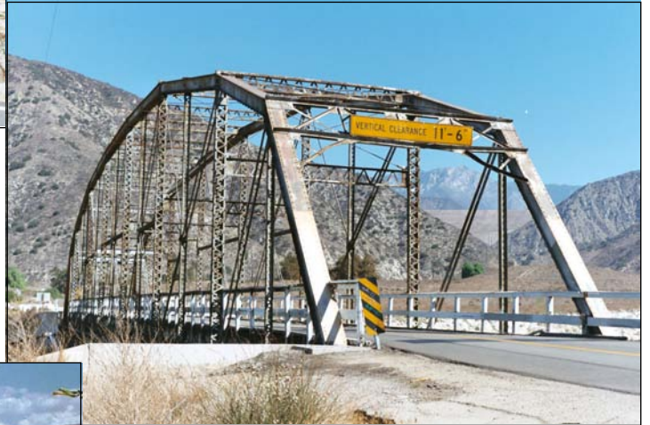
Greenspot Bridge Over the Santa Ana River
