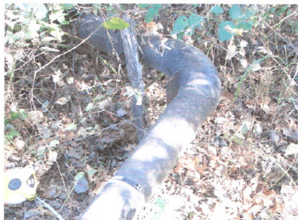
Remnant Steel Pipe at End of Retaining Wall
