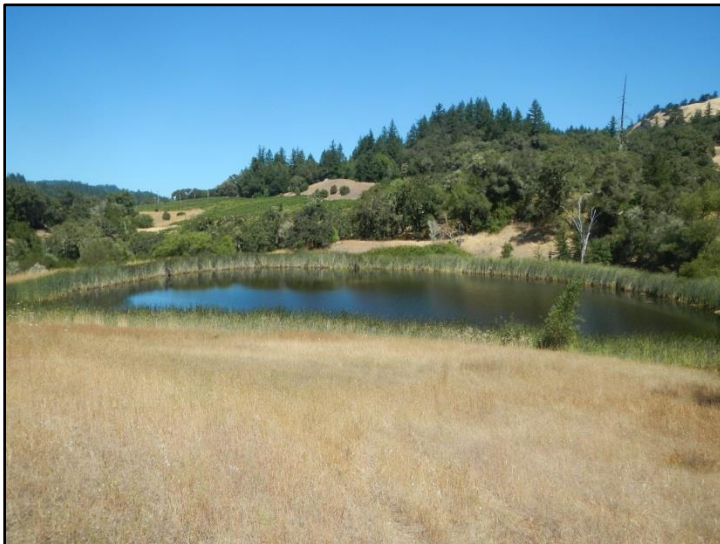
Figure 4. Construction of Reservoir 1 has resulted in substantial changes to the bed, bank and channel of a stream, which does not comply with FGC section 1602. The reservoir can interrupt natural stream processes, including transport of sediment and benthic macro-invertebrates downstream. Placement of earth materials into a stream channel from construction of the dam has resulted in
