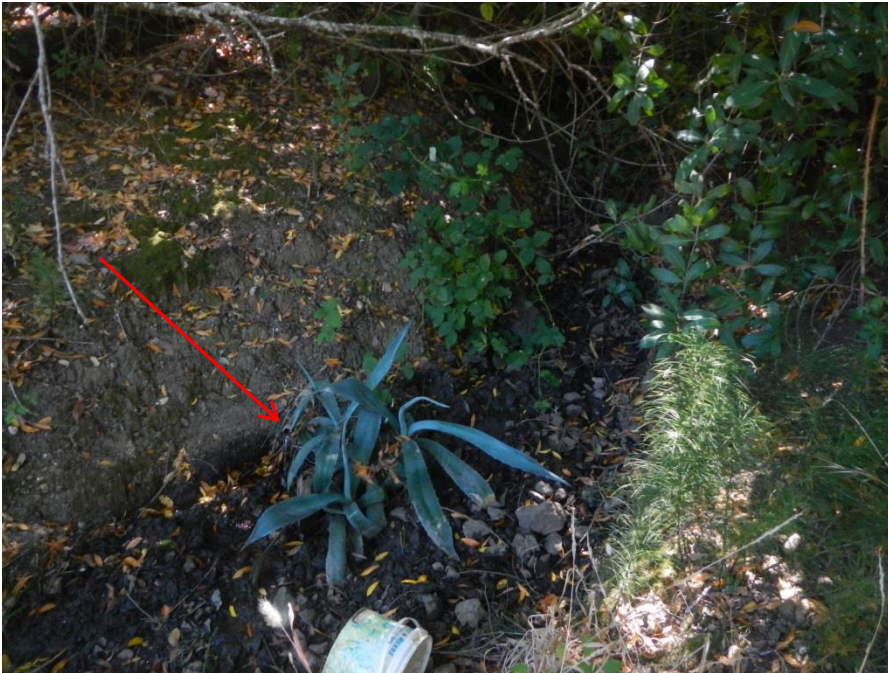
Figure 8. A small pipe is shown by the red arrow that was described as being connected to a horizontal well. Seepage within the stream channel upstream the pipe indicates not all of the surface flow in the stream can be attributed to water from the pipe.
