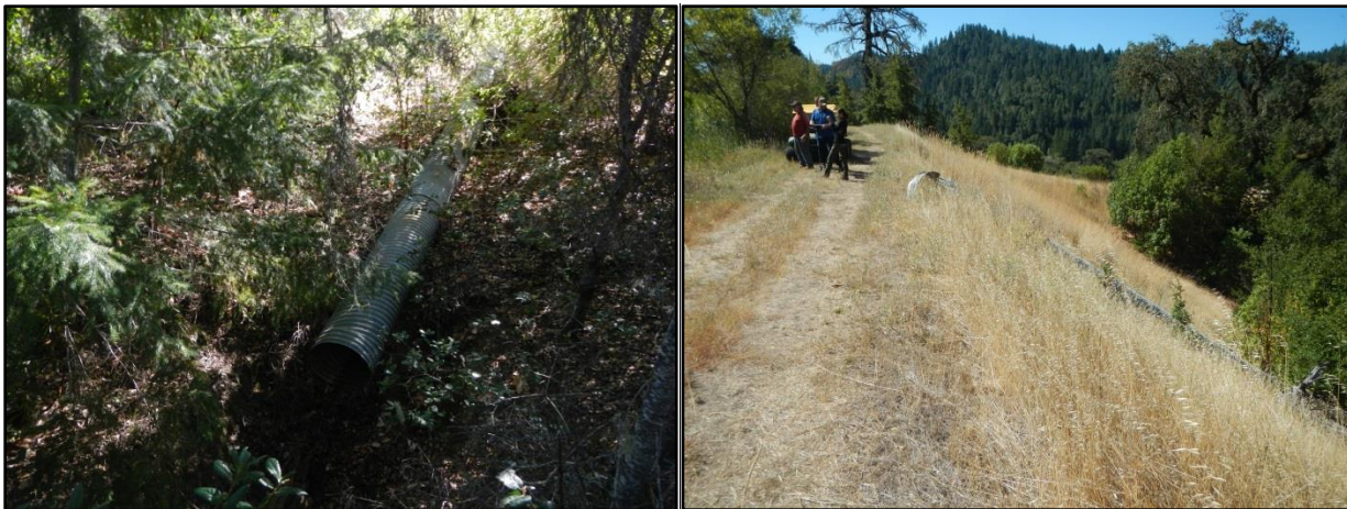
Figure 3. The dam obstructs the natural surface flow of a stream and only allows bypass flows at times when the reservoir spills, see FGC sections 1602 and 5937. Placement of earth materials into a stream channel from construction of the dam has resulted in placement of deleterious sediment where they can enter waters of the state, which does not comply with FGC section 5650.
