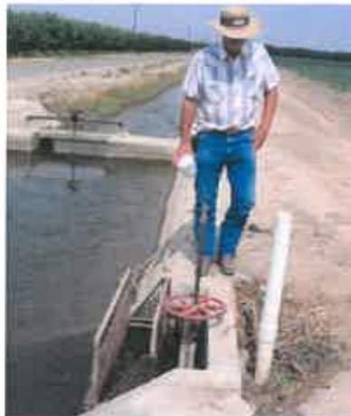
Figure B-10. This stilling well is properly located, but it has too small a diameter. The operator also needs to know the elevation difference between the top of the stilling well and the gate frame, which requires an extra computation to determine the difference in head across the gate.
