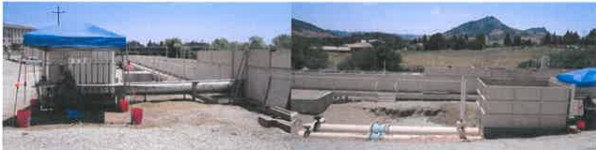
Figure B-2. ITRC gate calibration facility
