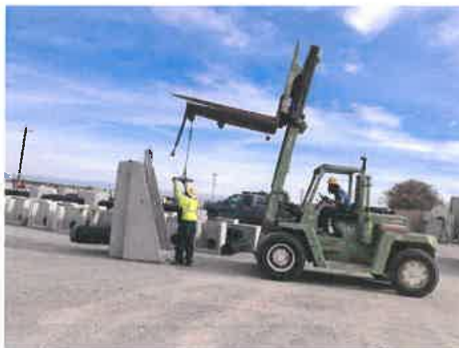
Figure B-14. Pre-cast metergate ready for transport
