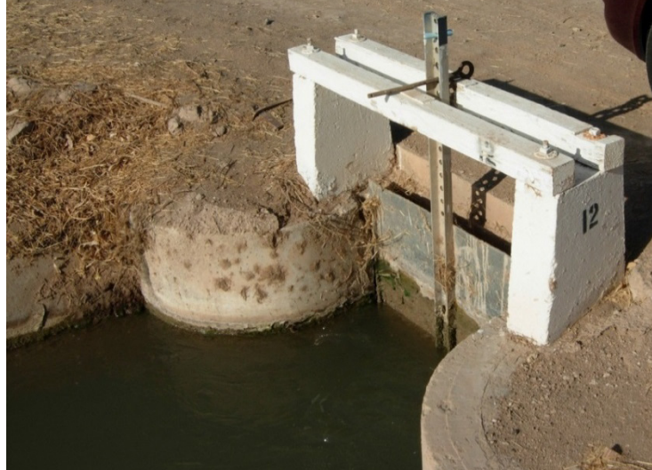
Figure 2. A typical IID jack gate
