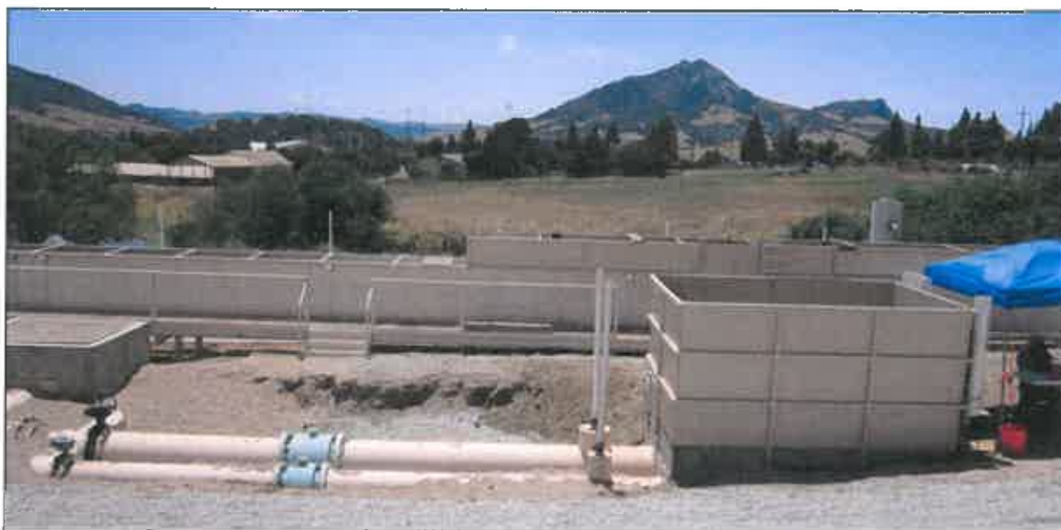
Figure A-6. Completed testing setup after construction.
