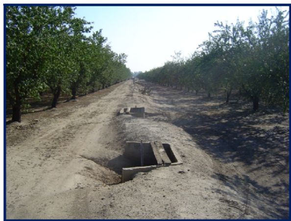
Figure 3-8. Surface Irrigation Valves
