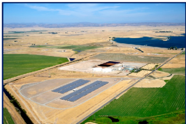
Figure 3-10. Nick C. DeGroot Water Treatment Plant and Robert O. Schulz Solar Farm
