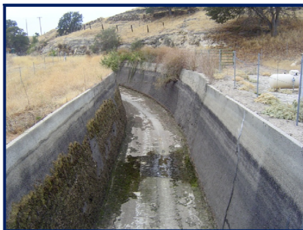
Figure 3-3. SSJID Upper Main Supply Canal
