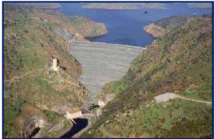
Figure 1-1. New Melones Dam
