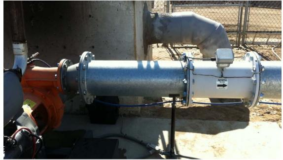
Figure A-5. Magnetic flow meter on delivery at Ra81.
