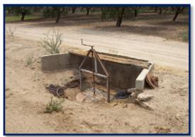
Figure 3-14. Orchard Valve Installed on SSJID Pipeline
