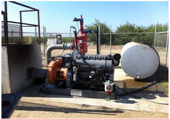
Figure A-1. Pump turnout on a District pipeline.
