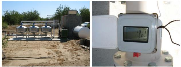
New Pump and Filter Station and Magnetic Flowmeter.
