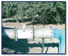
Figure 3-16. Magnetic Flow Meter
