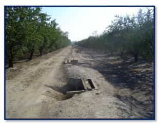
Figure 3-8. Surface Irrigation Valves
