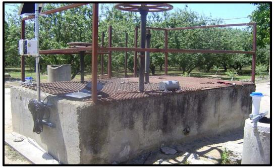
Figure A-3. Orifice gate turnout in a concrete box on a District pipeline.
