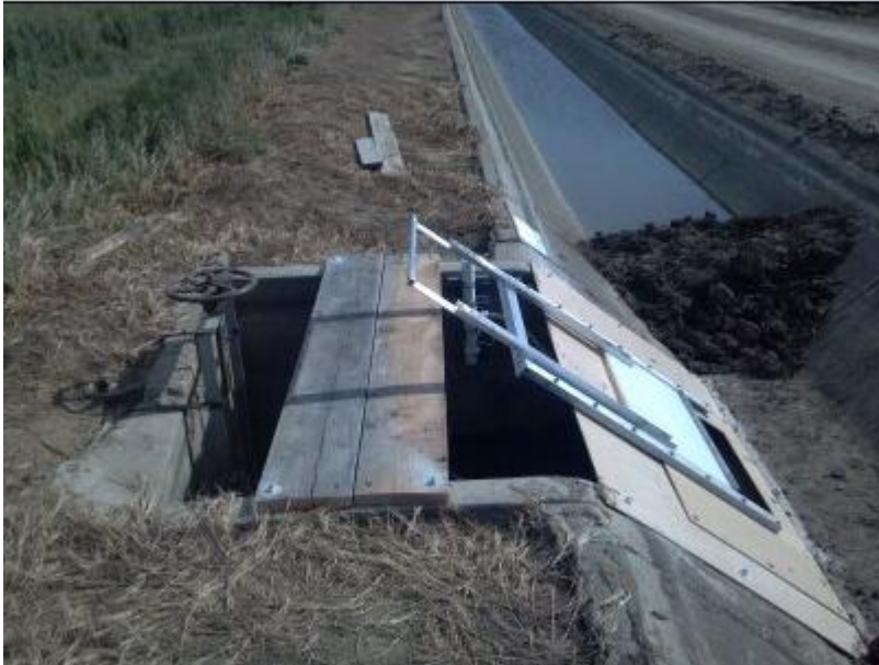
Figure 7.2: Fixed Orifice Plate
