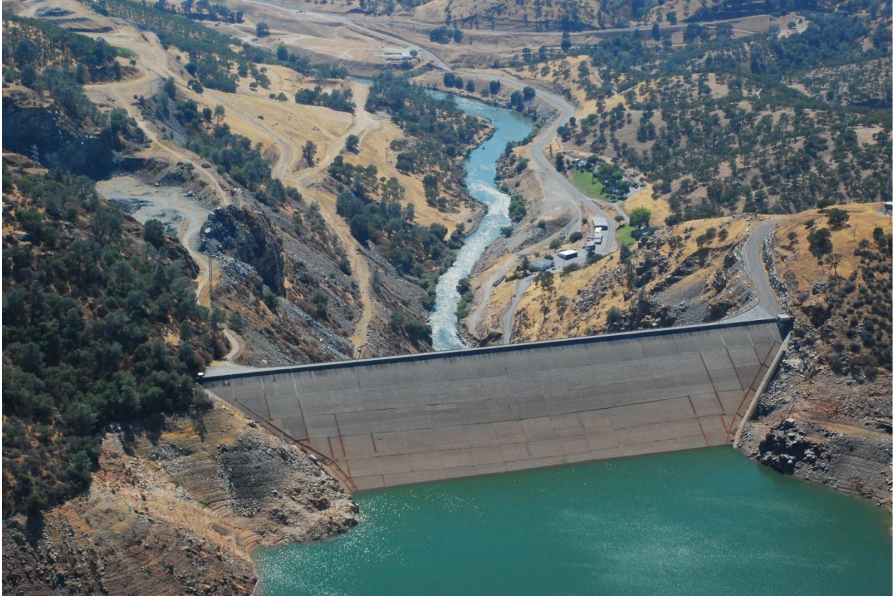
New Exchequer Dam
