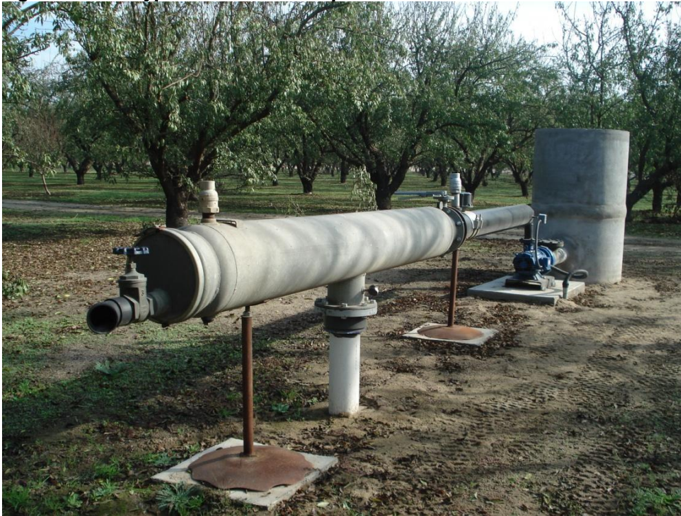
Figure F-4 Typical Booster Pump Installation
