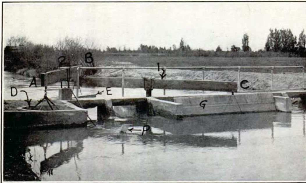
-AUTOMATIC CHECK GATE, TURLOCK IRRIGATION DISTRICT, CALIFORNIA.
