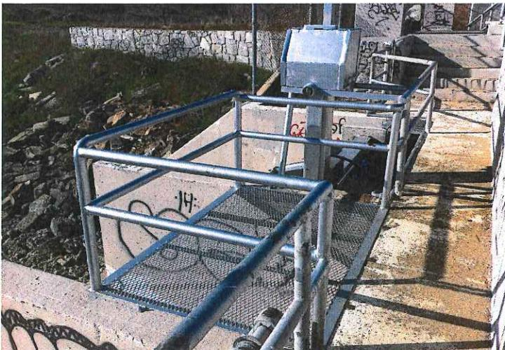
Above: Top view of new safety railing, catwalk, and vandalism protection enclosure
