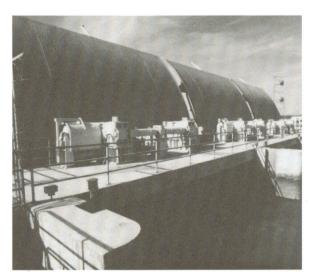
The Suisun Marsh Salinity Control Gates began operating in 1989. Each of the three gates measures 36 feet wide by 28 feet high and operates electronically to improve water quality in the marsh.
