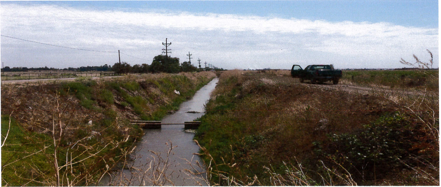
Photo 2: Photo looking east along the drain that borders Bethany Road within the WSID boundary. The drain collects tailwater which then flows back into Old River Cut.
