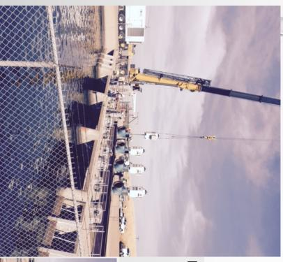
Installation of the temporary pumping plants the capacity of these plants At Check 10 355 CFS At Check 7 210 CFS At Check 4 140 CFS
