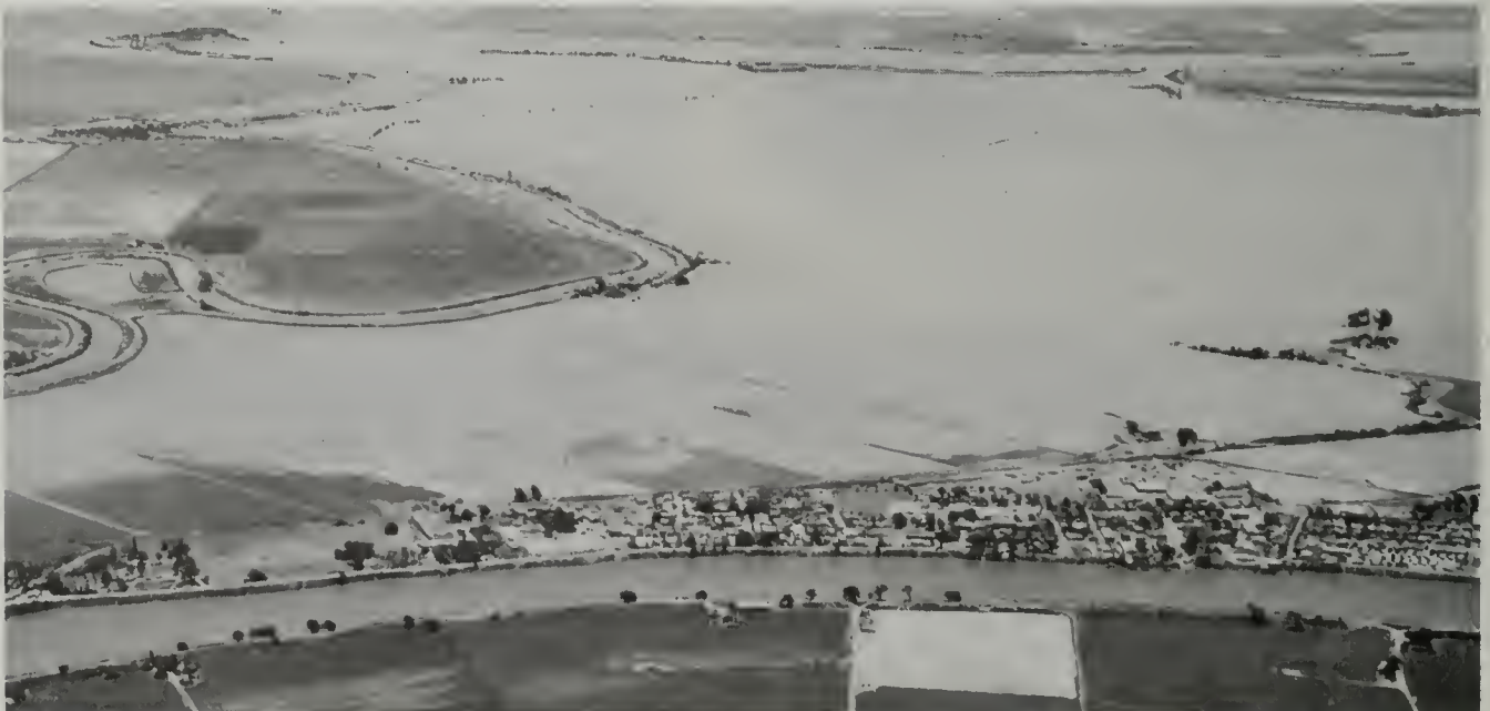
The Brannan-Andrus flood of June 1972 was caused by the failure of a section of levee along the San Joaquin River.
