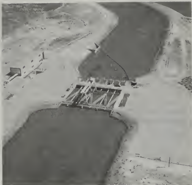
Fish screening facilities at the intakes to the SWP Delta (left) and CVP Tracy (right) Pumping Plants. With water in the adjacent channels flowing toward the export pumps, fish have a difficult time avoiding the pumping plants and must be screened out. Large fish are screened out completely but the louvre screens are not as efficient in screening small fish. Those that are screened out are collected and transported in tank trucks to the western Delta. Some of those not screened survive and grow to adulthood to form a significant fishery in the aqueduct systems as shown below.
