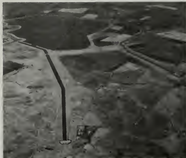
Clifton Court Forebay serves as the main Delta diversion point for the SWP. The Tracy Pumping Plant pumps water directly from Old River into the CVP Delta-Mendota Canal.
