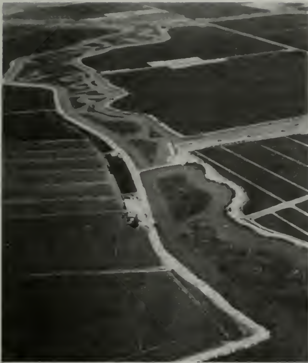
Disappointment Slough looking west near where the Peripheral Canal will cross. The first stage of the canal, which will be siphoned under the slough, will terminate just south of here. Water from the Peripheral Canal will be released into Disappointment Slough and other sloughs along the canal route to improve the water quality.
