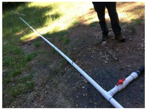
Photo 3 (POD1): Percolating GW Well - waterlines outlet of groundwater well.
