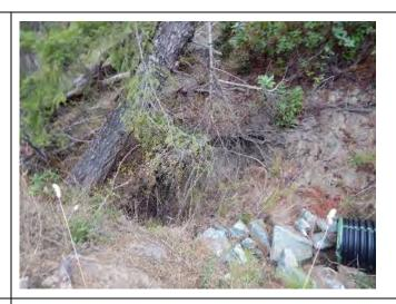
Photo 36: Image of downstream side of stream crossing C2 showing streambank erosion and stream bed armoring.
