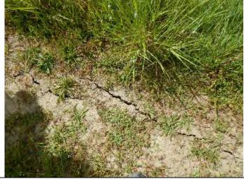
Photo 12: Image of surface cracking within top of POND2 berm
