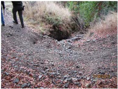
**Figure 1.** Substantial obstruction of the natural flow and alteration of the bed, bank, and channel of an unnamed tributary to Bear Creek and the South Fork Eel River by the construction and use of a wet ford crossing. This feature is causing erosion of road and bank delivering sediment to Waters of the State.
