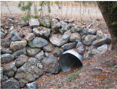
**Figure 9.** Substantial obstruction of the natural flow and alteration of the bed, bank, and channel of an unnamed tributary to Bear Creek and the South Fork Eel River by the placement of a culvert and fill within the channel.
