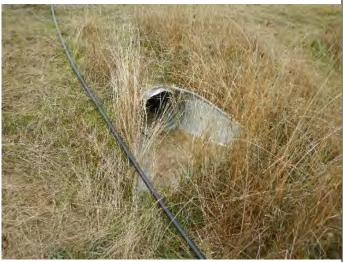
Photo 8: Closer view of POND1 outflow pipe (OUT1) with a layer of sediment covering the bottom of intake.
