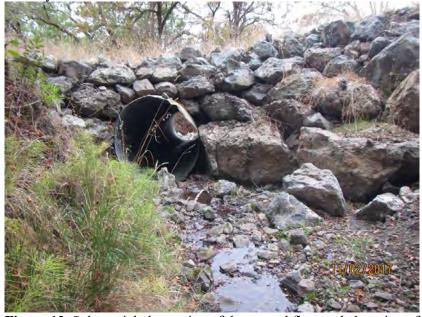
**Figure 12.** Substantial obstruction of the natural flow and alteration of the bed, bank, and channel of an unnamed tributary to Bear Creek and the South Fork Eel River by the placement of a culvert and fill within the channel.
