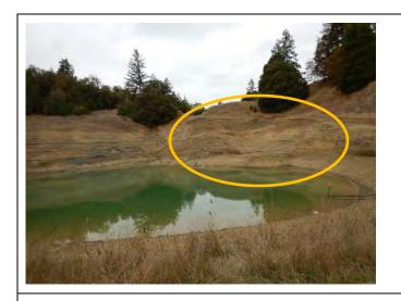
Photo 3: View uphill of upper pond (POND1) from earthen berm. Landslide into pond seen on right side of image (see orange circle).
