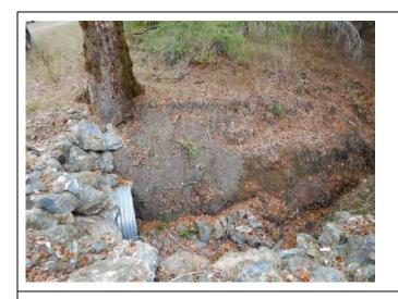
Photo 43: Image of upstream side of stream crossing C3 showing erosion of streambanks and armoring of streambed.
