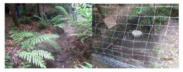
**Figure 18.** Substantial obstruction of the natural flow and alteration of the bed, bank, and channel of an unnamed tributary to Bear Creek and the South Fork Eel River for water diversion by diverting the natural flow to an impoundment and then diverting water from a cistern located in the center of the impoundment.
