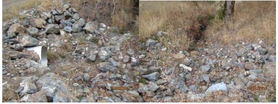
**Figure 8.** Substantial obstruction of the natural flow and alteration of the bed, bank, and channel of an unnamed tributary to Bear Creek and the South Fork Eel River by the placement of a culvert and fill within the channel.
