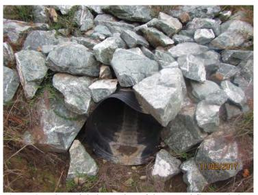
**Figure 2.** Substantial obstruction of the natural flow and alteration of the bed, bank, and channel of an unnamed tributary to Bear Creek and the South Fork Eel River by the placement of a culvert and fill within the channel.
