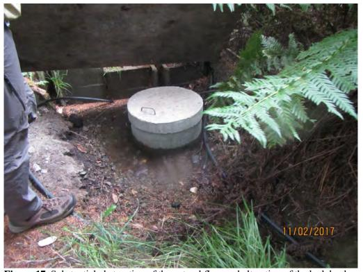
**Figure 17.** Substantial obstruction of the natural flow and alteration of the bed, bank, and channel of an unnamed tributary to Bear Creek and the South Fork Eel River for water diversion by impounding the channel with concrete and diverting water from a cistern located in the center of the channel.
