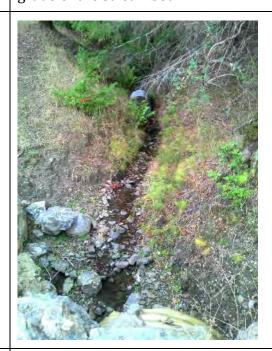
Photo 50: Image of downstream side of stream crossing C6 showing culvert was not placed in alignment with the Class II stream channel.
