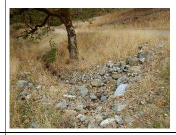
Photo 46: Image of downstream side of stream crossing C4 showing armoring of streambed and banks.
