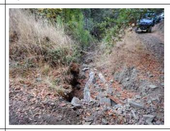
Photo 34: Image of downstream side of stream crossing C1 blocking Class III watercourse and showing erosion of the streambank.
