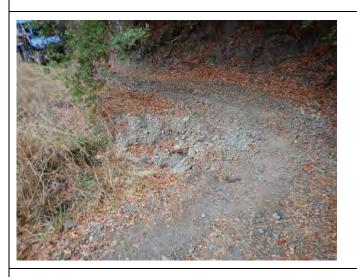
Photo 33: Image of ATV stream crossing C1 blocking Class III watercourse located approximately 28 feet from outdoor cultivation area CA2.
