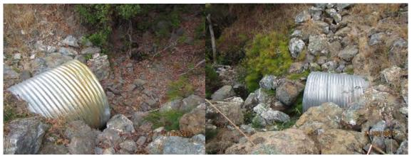
**Figure 13.** Substantial obstruction of the natural flow and alteration of the bed, bank, and channel of an unnamed tributary to Bear Creek and the South Fork Eel River by the placement of a culvert and fill within the channel.
