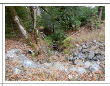
Photo 44: Image of downstream side of stream crossing C3 showing armoring of streambed and streambank.
