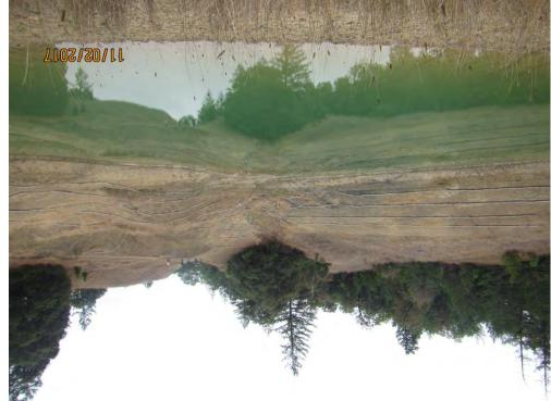
Figure 5A. Substantial discharge of sediment to Waters of the State from unpermitted grading and pond construction that removed vegetation and triggered slope instability leading to land sliding into the pond and then into the on stream pond.
