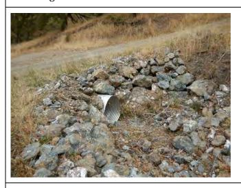
Photo 45: Image of upstream side of stream crossing C4 showing armoring of streambed and banks.
