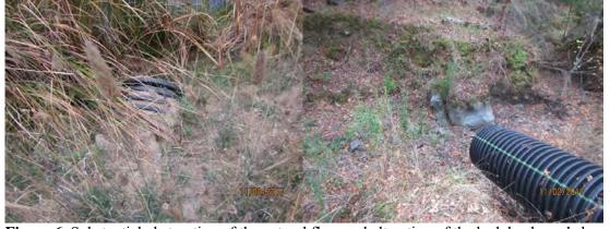
**Figure 6.** Substantial obstruction of the natural flow and alteration of the bed, bank, and channel of an unnamed tributary to Bear Creek and the South Fork Eel River by the placement of a culvert and fill within the channel.
