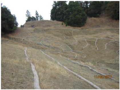
**Figure 5B.** Substantial discharge of sediment to Waters of the State from unpermitted grading and pond construction that removed vegetation and triggered slope instability leading to land sliding into the pond and then into the on stream pond.
