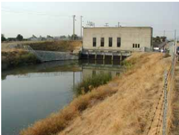
Contra Costa Canal Pumping Plant No. 1 near Oakley
