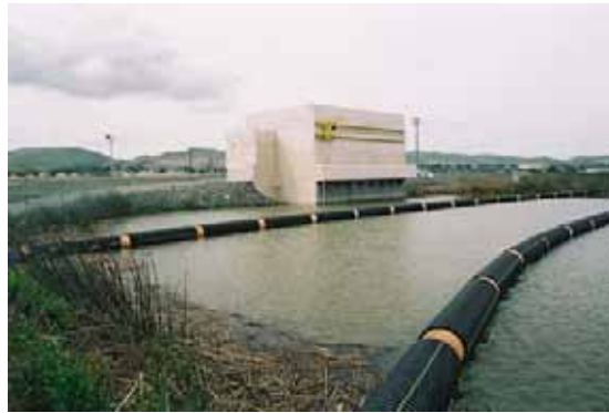
Contra Costa Water District's Mallard Slough Pumping Station, west of Pittsburg, is only used after periods of high Delta outflow when the water in Suisun Bay near Chipps Island is fresh enough to meet CCWD's delivered chloride goal.
