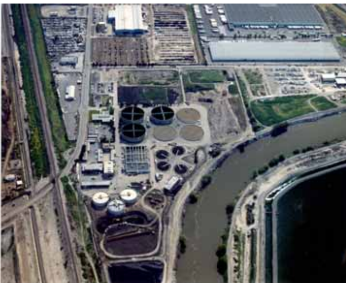
The City of Stockton's 48-million-gallon per-day Regional Wastewater Control Facility, located beside the San Joaquin River just north of Highway 4.
