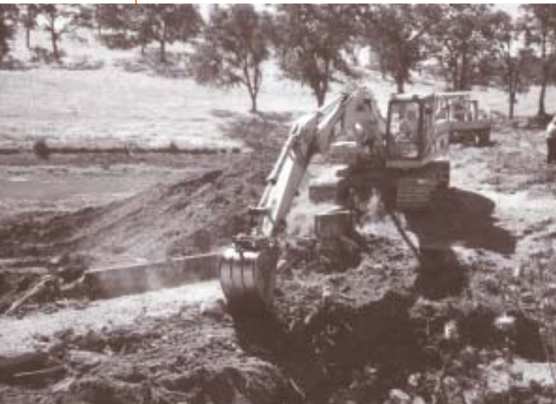
Bulldozer removes a dam on Murphy Creek.
