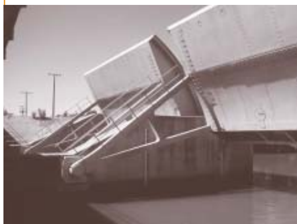
Delta Cross Channel Gates
