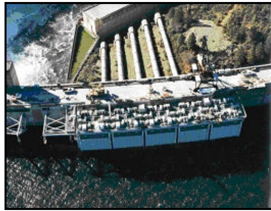
Shasta Temperature Control Device, Dam, and Powerplant. The five TCD bays are on the right center, and the low-level intake support structure is on the left.
