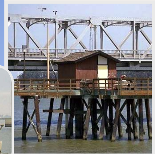
Shore-based continuous monitoring
