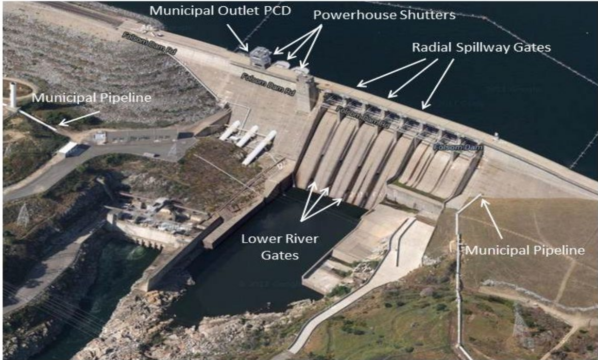
Appendix G4 Figure 1. Folsom Dam Outlet Structures (Google Maps, 2013)
