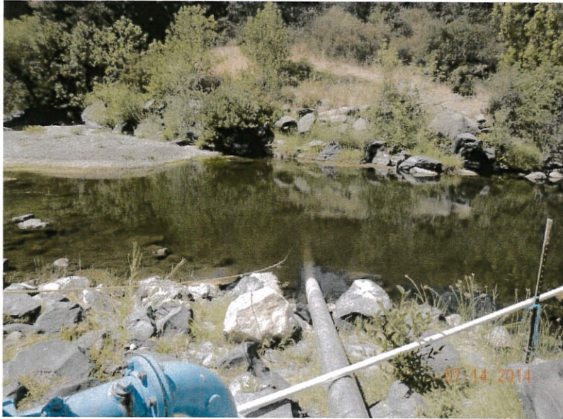
Photo 14 – Diversion upstream of USGS gage
