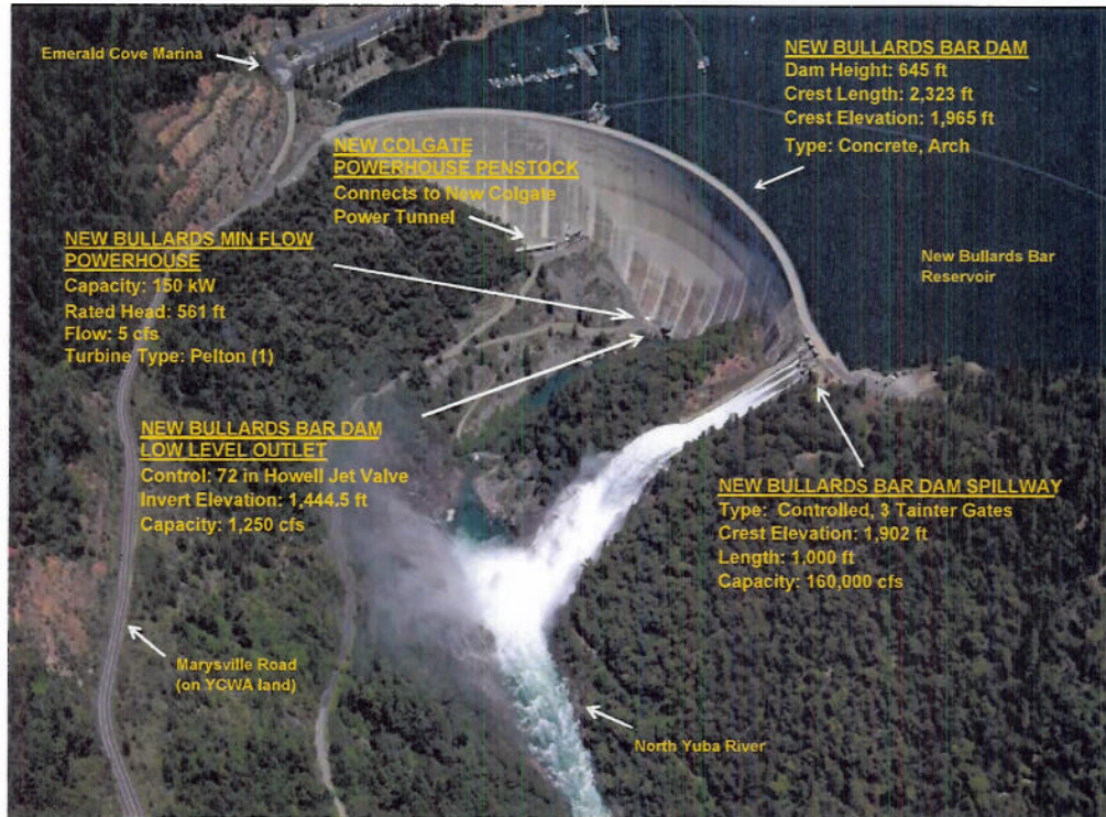
Figure 3.1-3. New Bullards Bar Dam and New Bullards Bar Minimum Flow Powerhouse.
