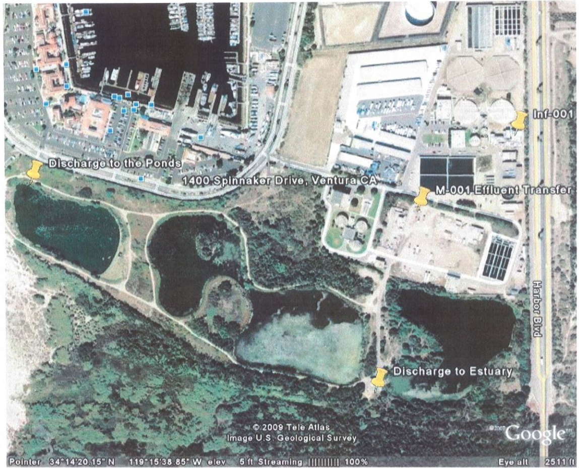
Figure 5: Ventura WRF Discharge Location Photos
