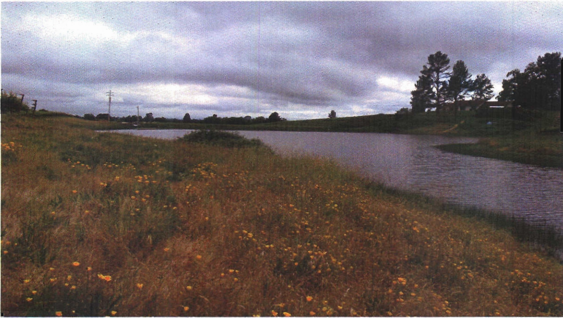
Upstream of Reservoir looking downstream at dam
