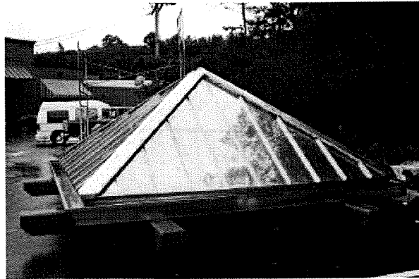
Copper roof section, prior to installation
