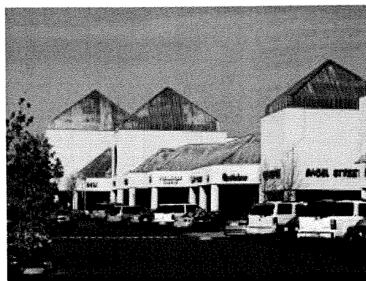
Copper roof, Redwood Shores California
