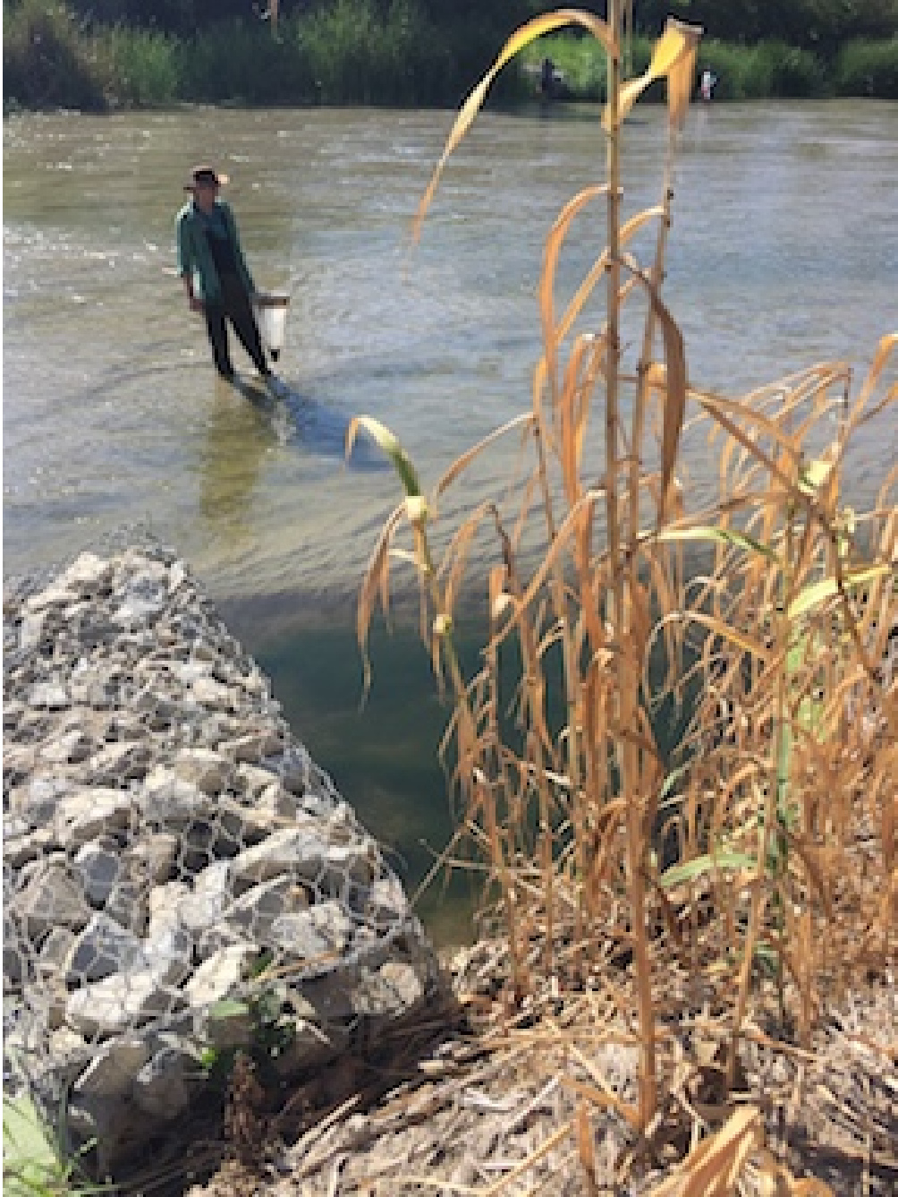
Figure 1. Gabion at bottom left of picture. Note the deeper water to the right, which is downstream of the gabion.
