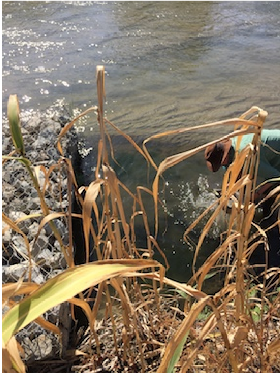
Figure 2. Gabion at bottom left of picture. BMI samples were taken 1m downstream of the gabions.
