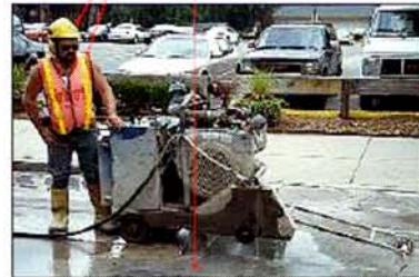
Correct PPE, but no control of sediments
