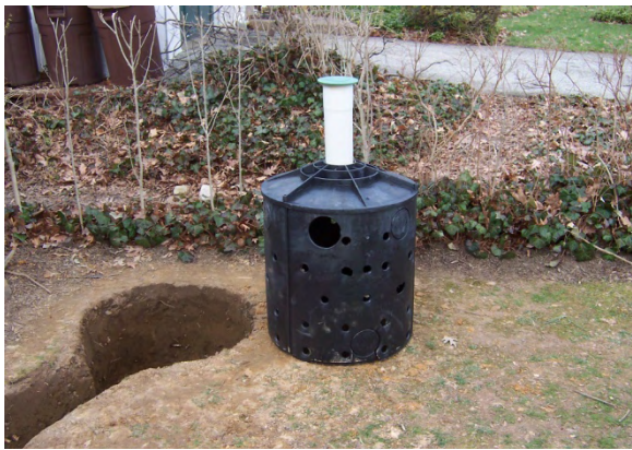
Drywell installation
