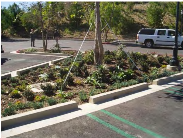
Bioretention in Parking Lots
