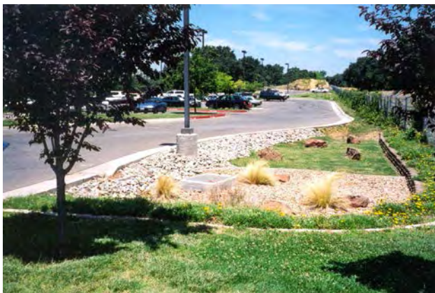
Sand filters connected to impervious surfaces
