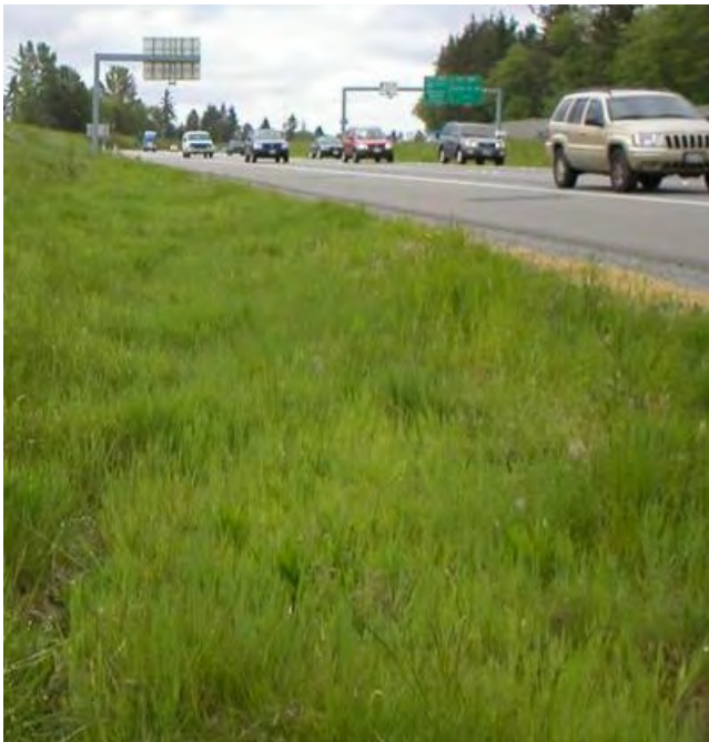
Vegetated filter strip captures runoff from freeway
