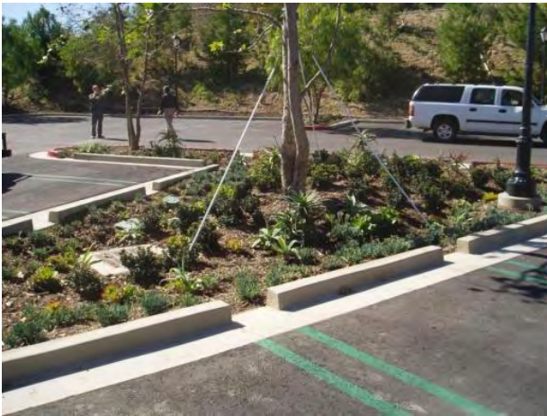
Bioretention in Parkway and parking lots
