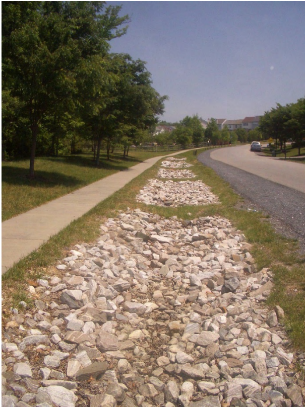
Rural Highway Infiltration Trench
