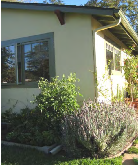
Diverted Roof Runoff City of Santa Barbara
