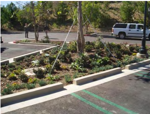
Bioretention in Parkway and parking lots
