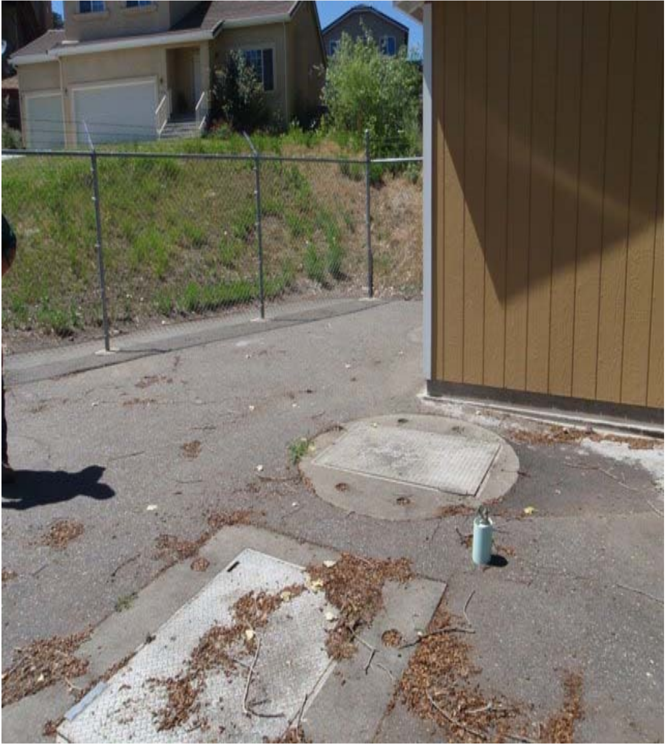
Photo 11: Debris on riverview lift station grounds and on the wet well cover
