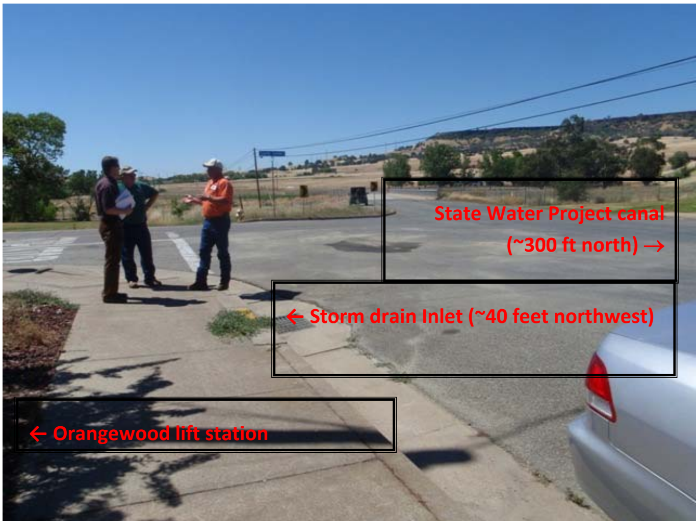
Photos 14: Orangewood lift station near storm drain inlet and California State Water Project surface water canal
