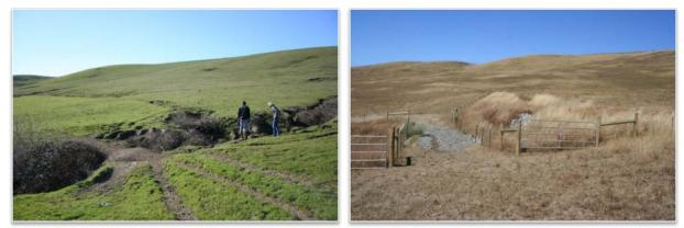
Figure 15: Pre-construction photo, left (2/2013) and post-construction photo, right (6/2015). The preconstruction photo shows a view of a livestock culvert crossing and active side gully headcutting. The postconstruction photo shows a riparian fence encompassing the gully headcut and bordering a livestock culvert crossing repair.
