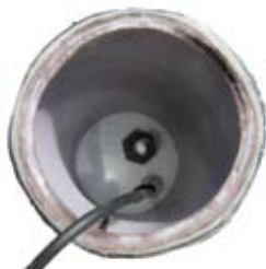
One or 50 micron pre-filter keeps sediment away from the pump.
