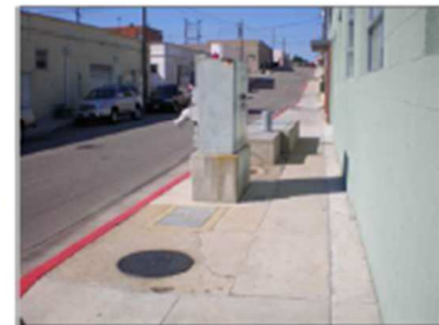
Lift Station #2, El Segundo, CA
