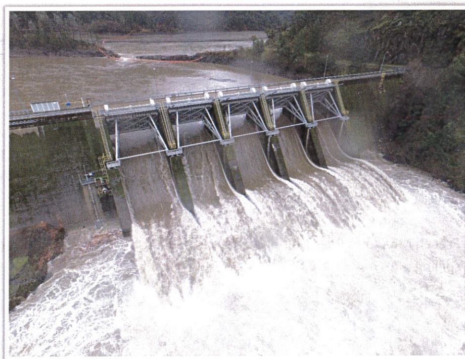
Ralston Afterbay dam with all five gates open
