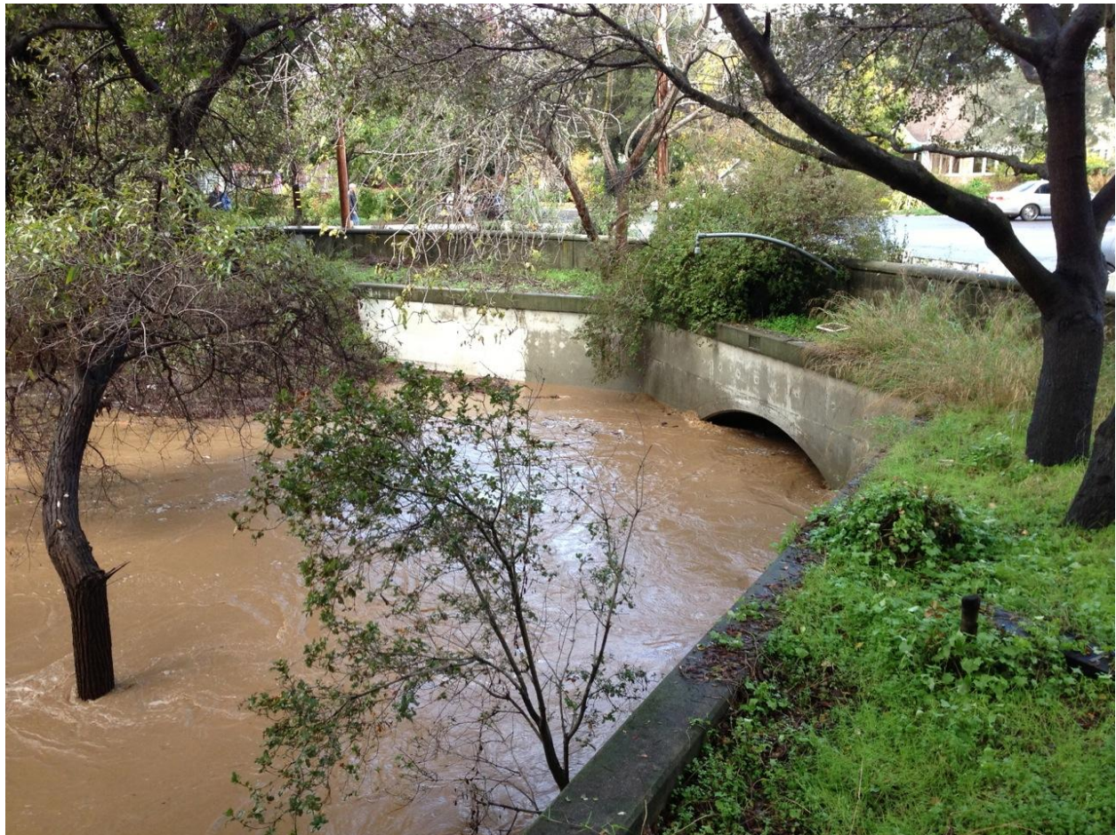
Figure 2 – Existing Culvert at Pope/Chaucer
