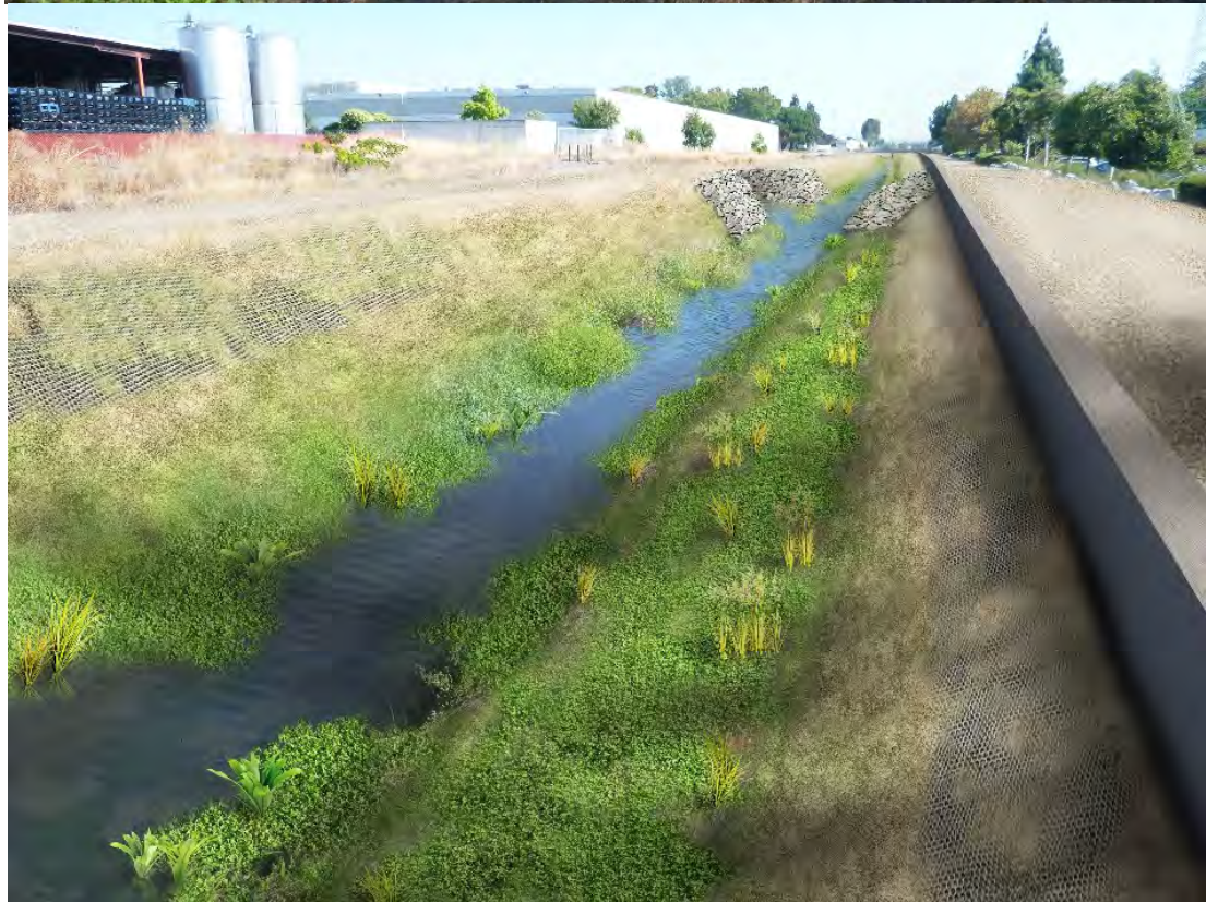
Figure 3.5 Photo-simulation A (Completed Project): Terraced Wetland, Floodwall, and confluence with Piedmont Creek
