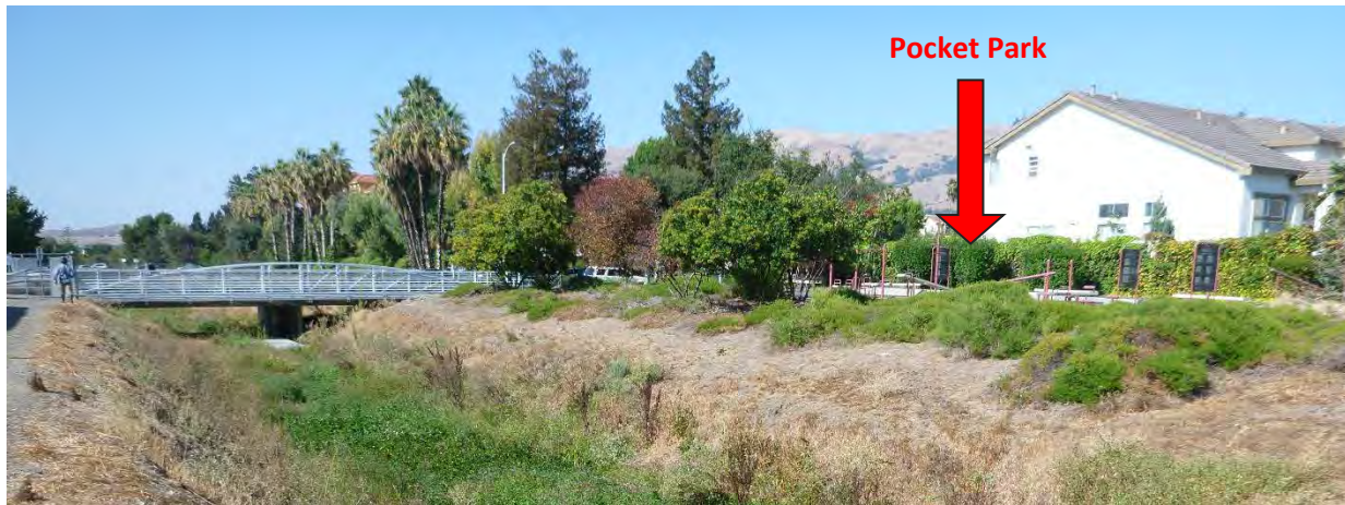
Figure 3.16 Looking Downstream toward Los Coches Street and Pocket Park
