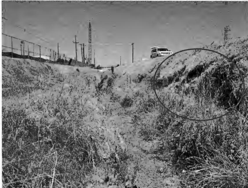
**Figure 3A:** Bank erosion upstream of Montague Expressway
