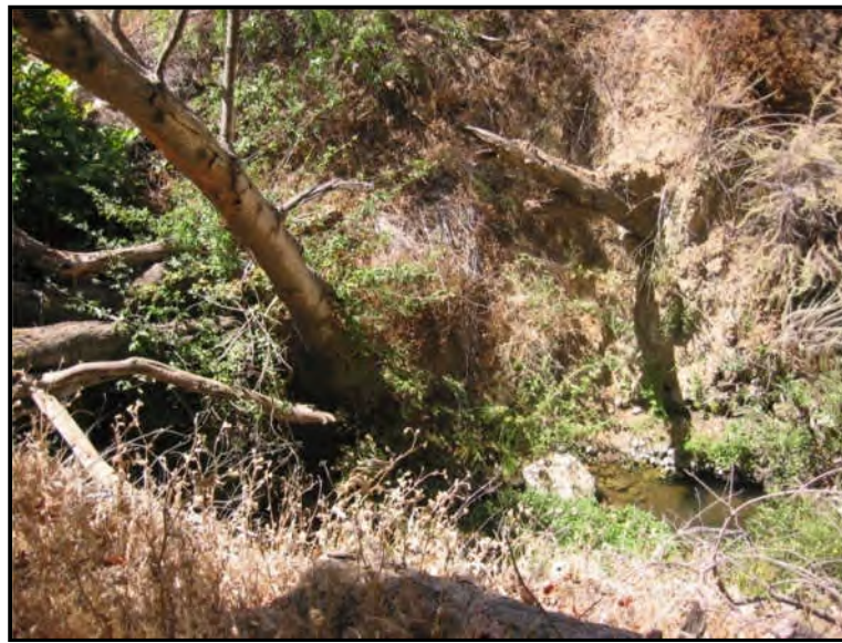
Photo 2.4 Mass Wasting Directly into Creek near Upstream Limits of Reach 4
