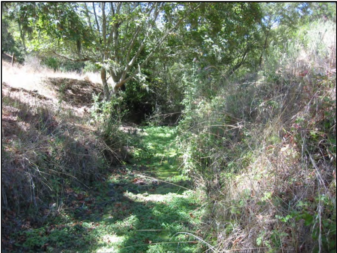
Photo 2.2 Typical Channel in Reach 2, Low Gradient
