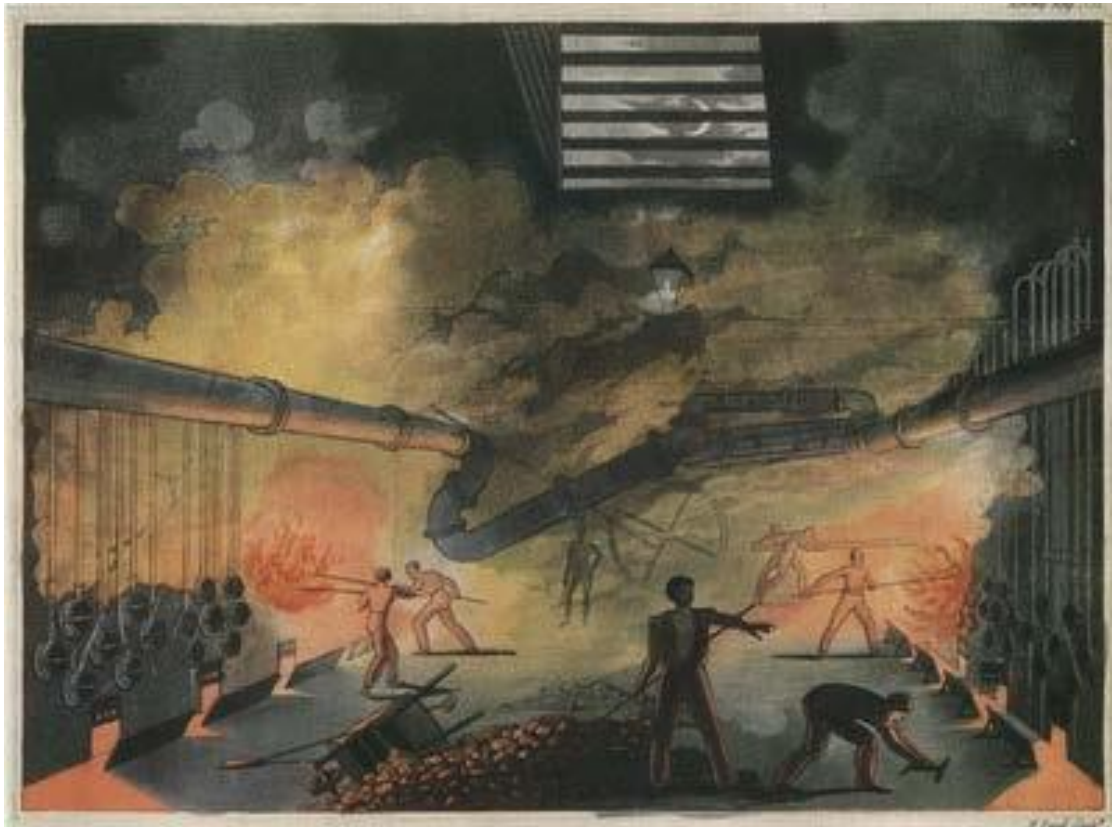
Figure 1. Drawing of the retorts at the Great Gas Establishment Brick Lane, from The Monthly Magazine (1821), conceptualizes 19th century manufactured gas plant operations.
