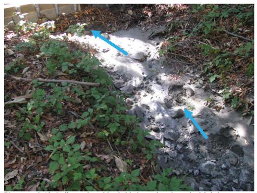
**Photograph 13**: Sediment deposition behind a trash and woody debris interceptor along the unnamed open drainage (9-18-2015 HTK)
