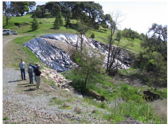
Nearer view of slide area showing head scarp adjacent to road, slide face, and base of slide in upland zone above creek.
