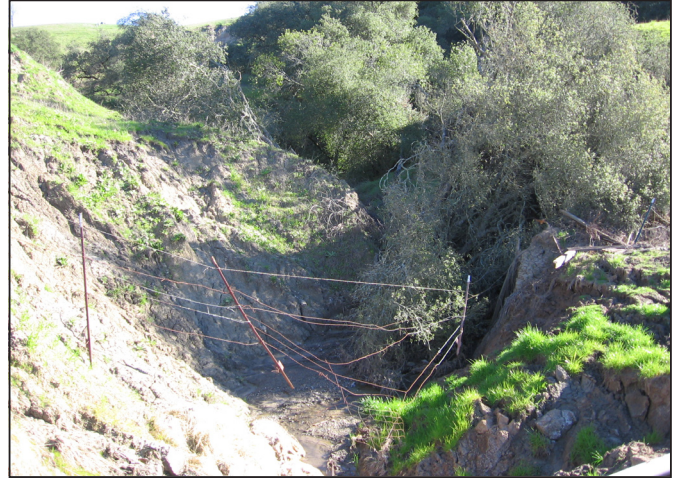
Photo b. Toe of active slide pushes eroded material directly into creek (Feb. 2006).
