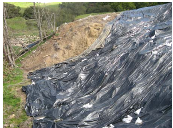
View of slide zone showing arcuate slide face in profile. Project treatments would include grading of slide face and strengthening toe of slide area with earthwork and tree plantings.
