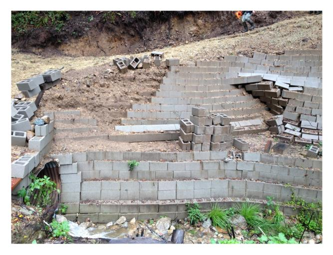
Outfall of Second Unauthorized Culvert and Failing Cinder Block Wall Within and Above Creek Bank
