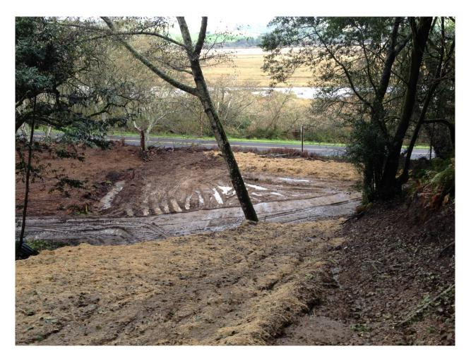
Road Slumping and Erosion from Unauthorized Grading
