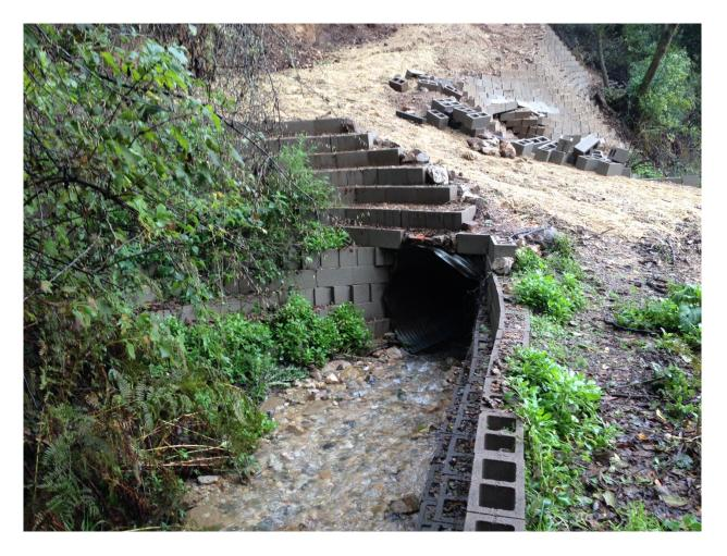
Invert of Second Unauthorized Culvert and Failing Cinder Block Wall Within and Above Creek
